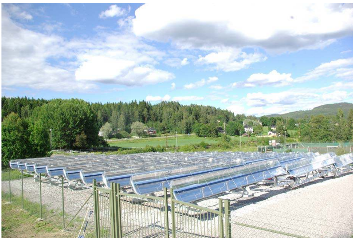
Figure 4. Absolicon's installation at Stödehuset is Sweden's largest hybrid installation with 400 m 2 of concentrating solar collectors. The plant produces 40 kW of electricity and heat to the adjacent sports hall and swimming pool. (Courtesy Joakim Byström)
