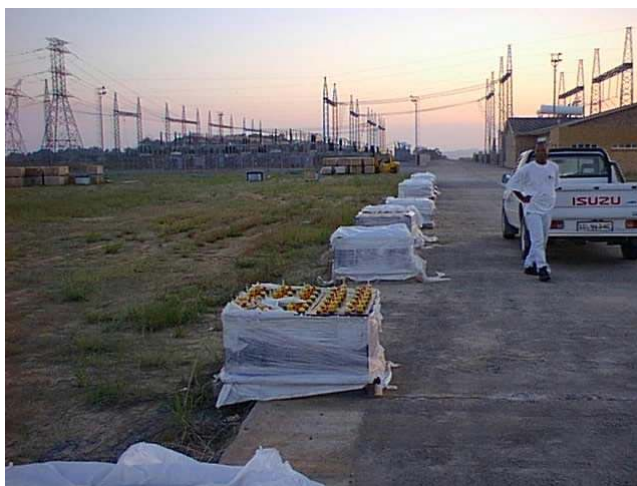
Figure 1: Incorrect storage of batteries
