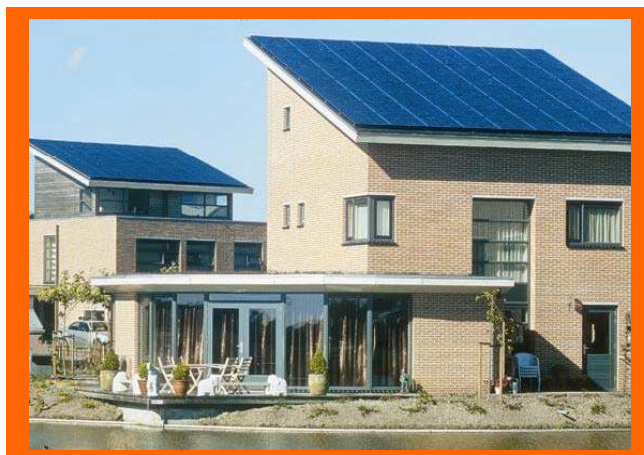
Figure 1 - 131 kWp Solar PV Community in The Netherlands (source: Bear Architecten)
