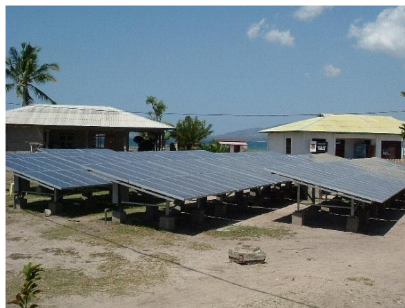
Figure 1: Pomelo, Indonesia, 24kWp, 20-kWh battery, 125-kVA genset (photo: TRANSENERGIE)
