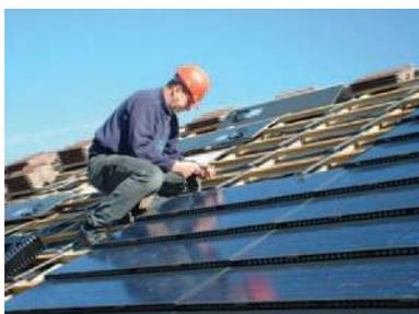
The roofers made the electrical connections between the modules as they progressed, using Multi-Contact (MC) connectors, which are touch-safe. The connections were made as straightforward as possible by installing the modules in columns to form a string from bottom to top. The strings comprised ten or twelve modules depending on the site. The PV contractor returned to test the continuity of the strings after the modules were installed and before the scaffolding came down.
