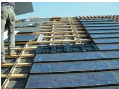
There were some minor problems with the PV-roof integration. For example, on the first completed roof, the roofer placed the felt between the counter battens and battens instead of underneath both, thus reducing the ventilation air gap. Emphasising the correct sequence of the counter battening here is crucial as this will be unusual practice to roofers.
