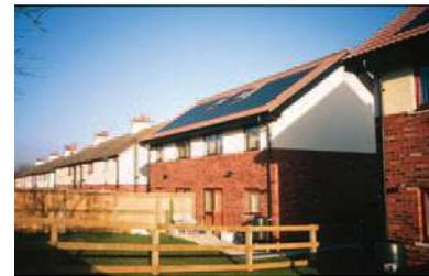
All roofs are at an angle of 35°. The PV tiles are designed to fit in with the conventional tiles' horizontal lines resulting in flushness with the roof. Also the contrast in colour between the red tiles and blue PV modules was deliberate. The overall result is an uncluttered roof with an eye-catching PV system.
