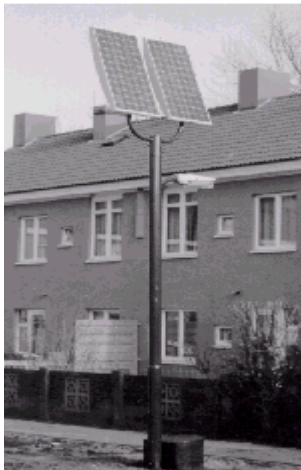
PV powered streetlight by Soluna Stroomwerk.
