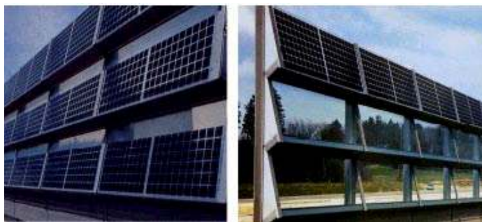
Different design of PV noise barriers: Type "zig-zag" by ARGE Crimmitschau (DLW Metecno)
