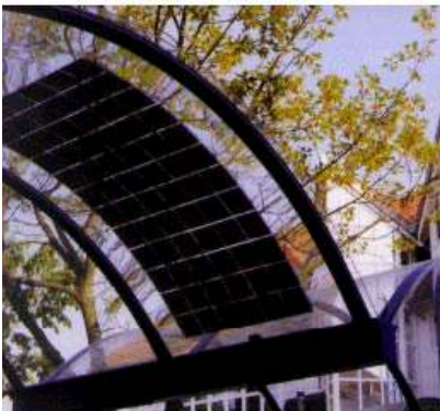
PV Bus-stop shelter with semi-transparent curved modules composed of polycrystalline cells. (Röhm)
