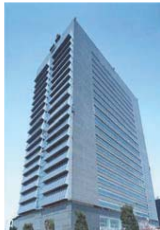
Figure 10: Commercial building with 214 kWp PV power incorporated in the skin of Kyocera headquarters in Kyoto, Japan. Source: Kyocera Corporation
