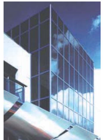
Figure 9: Industrial building with façade integrated PV system (8.4 kWp) at APS Photovoltaic Factory in Fairfield, California, USA. Source: DOE
