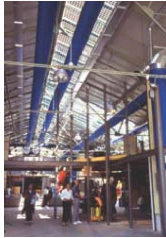
Figure 8: Children's Museum of Rome, Italy, with a semi-transparent canopy of 8.2 kWp solar power. Source: Abbate e Vigevano Architetti
