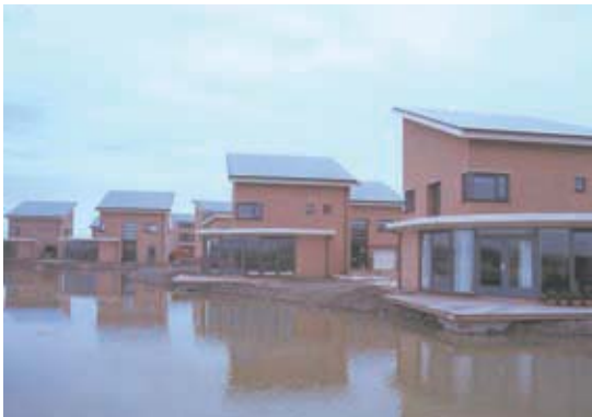
Figure 5: Langedijk solar and sustainable housing (some of the 2600 houses with 3775 kWp) in the Netherlands. Source: BEAR Architecten, photo: M. van Kerckhoven
