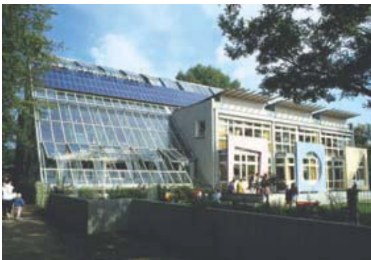
Figure 6: Children day care centre in Frankfurt, Germany with 10 kWp PV system positioned parallel to the glass house construction. Source: IEA PVPS T7 database
