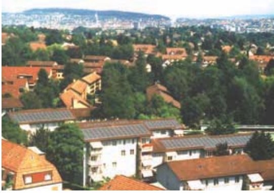
Figure 4: Marchwart project with roof integrated PV installation 53 kWp on multi-family buildings in a residential area of Zurich, Switzerland. Source: Enecolo
