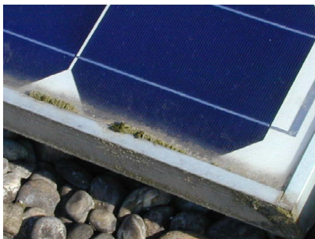
Fig. 14: Dirt accumulation above the frame (ewz).
