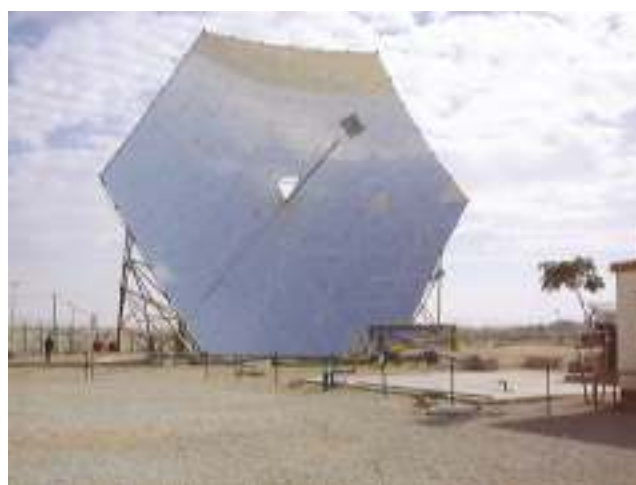
Figure B.12 The PETAL (Photon Energy Transformation and Astrophysics Laboratory) 400 m 2 aperture parabolic dish reflector at Sede Boqer (the square screen at its focal point is 1 m x 1 m in size)
