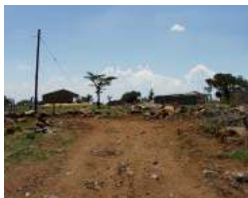
Electricity grid extension to a school
