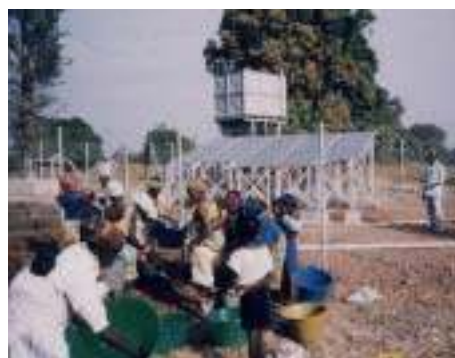
A PV powered water pumping system for a community in Mali.
