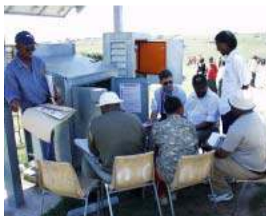
Training of field workers in South Africa on battery maintenance
