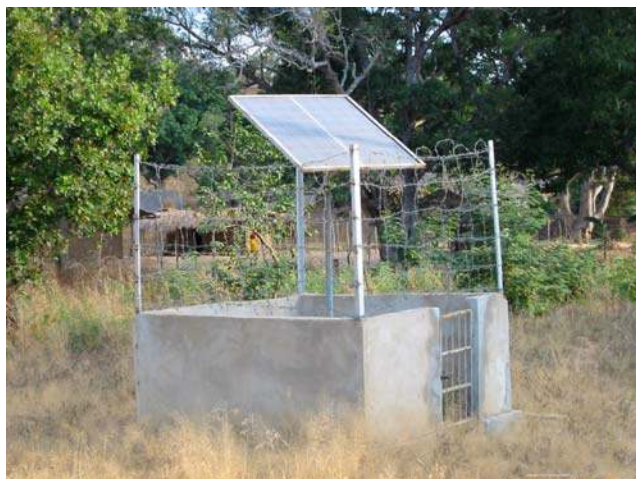
Security at Mecuburi, Mozambique
