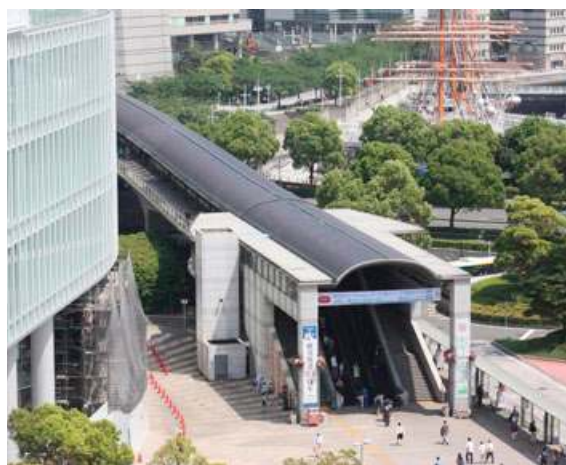
Minato Mirai 21 moving walkway PV System 79 kW, Yokohama City, Japan (Amorphous Silicon PV modules, Submodule by Fuji Electric, Module by Sanko Metal Industrial).
