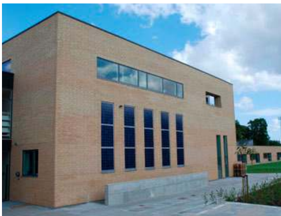
2.25 kW System integrated in the facade on the municipal school Slotsskolen, Horsens, Denmark
