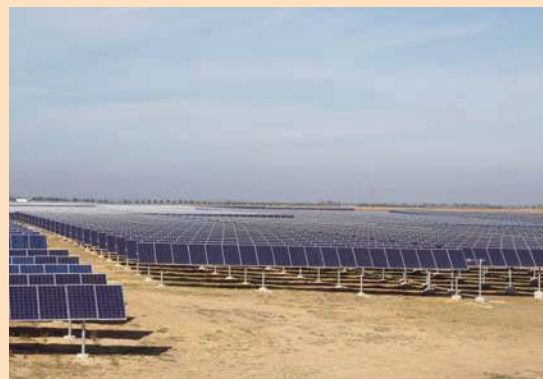
10 MW one-axis tracking c-Si Power Plant in Ferreira (photo Tecneira).
