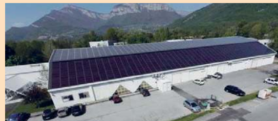
Figure 1 – PV System on a sport center in Challes les Eaux (Savoie Department) – 203 kW (Courtesy: Edisun Power)
