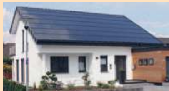
Roof integrated PV system with frameless CIGS tin film modules, courtesy of Wurth Solar / Germany
