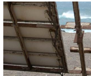
Fig. 12: Corrosion due to salt water [17].
