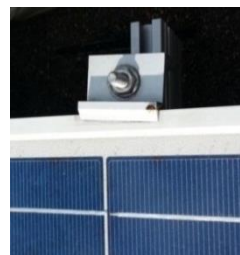
Fig. 20: Improperly installed end brackets [7]
