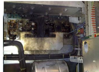
Fig. 7: Inverter failure due to an exploded insulated-gate bipolar transistor [4].
