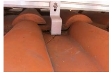
Fig. 19: Roof shingle has contact to roof tile [16].
