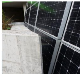
Fig. 11: Shading due to poor design [3].
