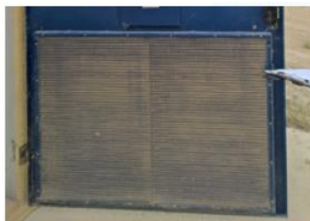
Fig. 6: A soiled air filter causes overheating 2 [3].
