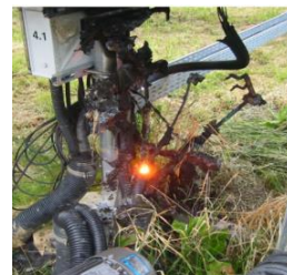
Fig. 4: A combiner box is destroyed due to fire [11]
