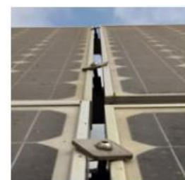
Fig. 21: Wrong combination of clamps and modules are used [3].
