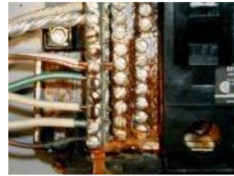
Fig. 7: Corroded interconnection, Image taken from Ref. [12].
