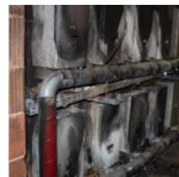
Fig. 3: Inverters are burned due to fire [8].
