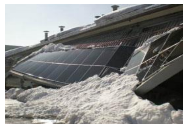
Fig. 15: Structural subsidence due to snow load [15].
