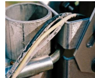
Fig. 31: Degraded cable insulation due to corrosion and mechanical stress [24].
