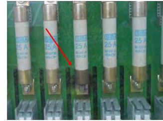
Fig. 28: Triggered string fuse [4].
