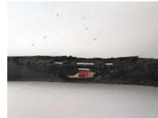
Fig. 29: Damage of cable due to rodent bite [22]
