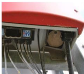
Fig. 5: A soiled air filter causes overheating 1 [3].
