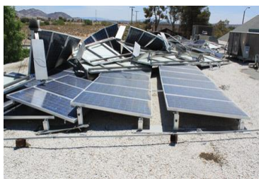
Fig. 13: Mounting system collapsed due to high wind load [13].
