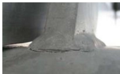
Fig. 14: Cracks due to mechanical stress [14].
