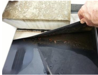
Fig. 18: Localized low spot for water [7].
