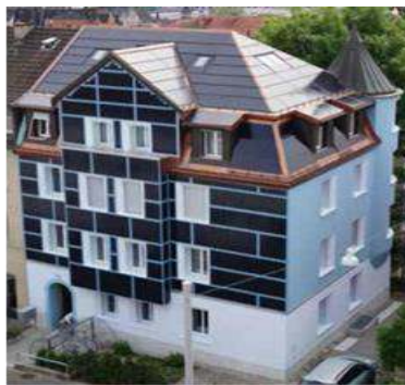
Photo of a building equipped with a complex BIPV system and its RADIANCE model, illustrating cases of partial shading [2].
