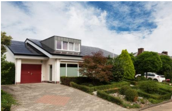
Figure 7: Example of a BIPV roof for a stand-alone house (renovation)
