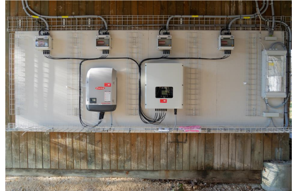
Multi-String PV inverters on the new test facility KNS of the PV LAB BFH-TI. 6 kWp (left) and 20 kWp (right).
