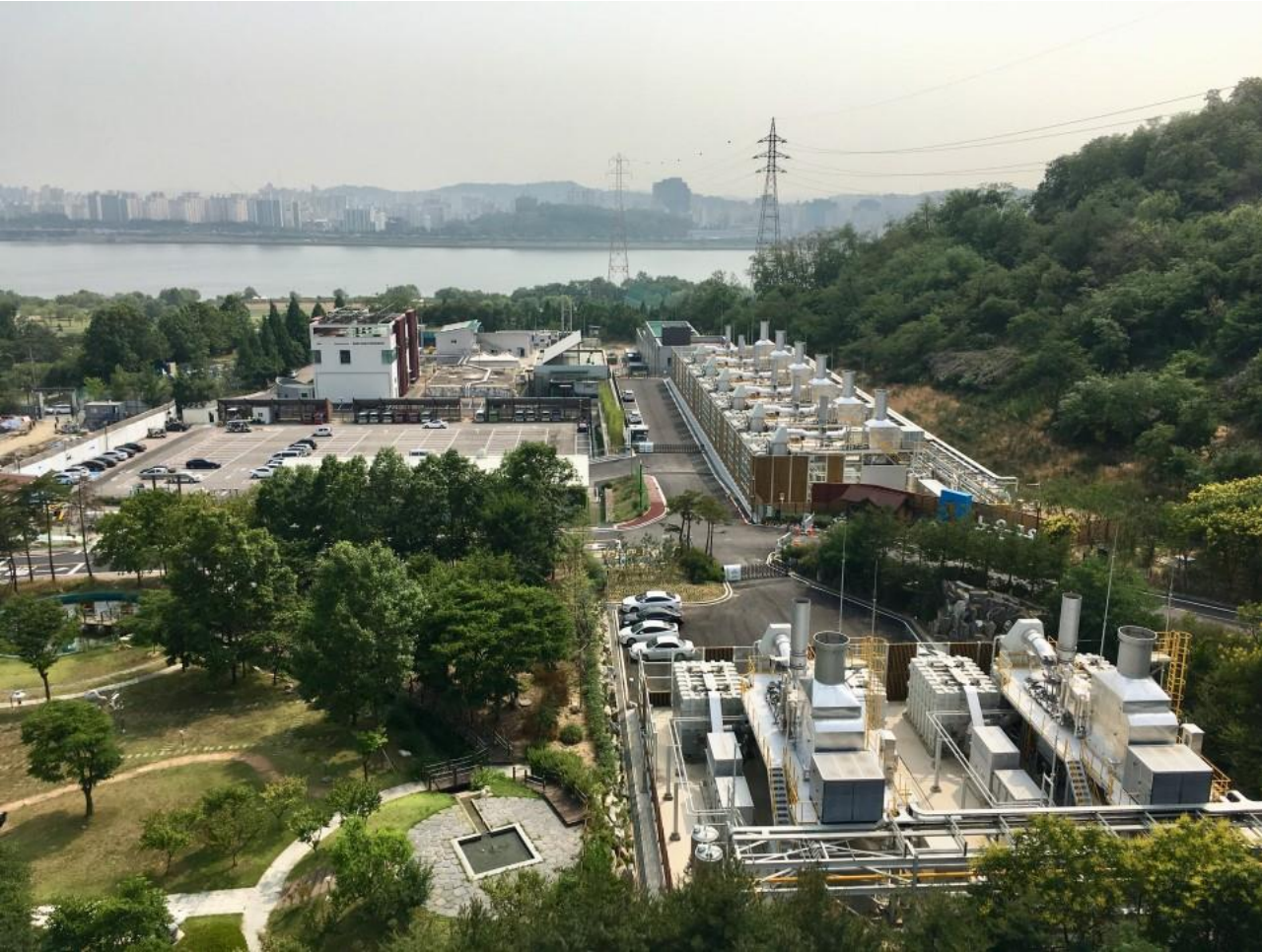
Seoul Noel Park (near World Cup Park) LNG Fuel Cell PJT (POSCO Energy)
