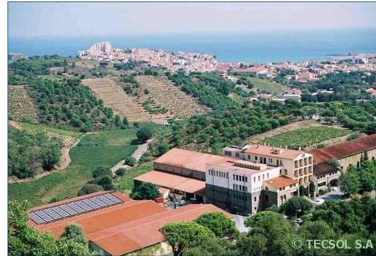
Banyuls vineyard solar cooling installation, France
