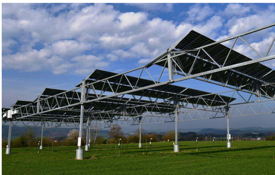
Figure 58: The pilot APV system uses bifacial glass-glass modules arranged in rows of two.
