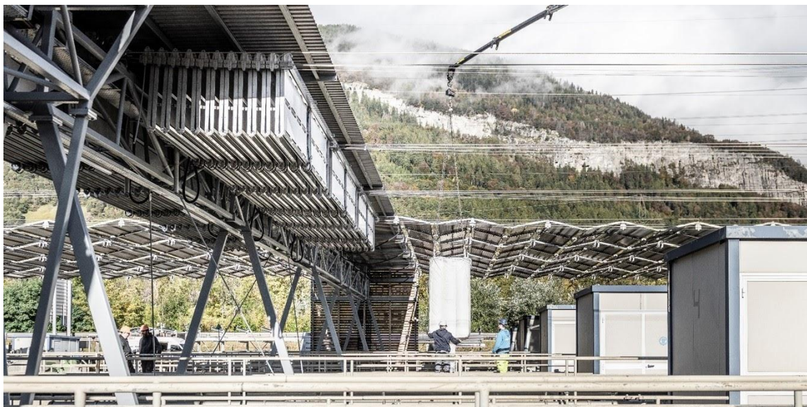
Figure 48: Parts of the PV foldable roof is opened to get access to regular service activities concerning the infrastructure of the wastewater treatment system (Source: dhp technology AG).
