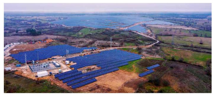
Fig. 1 - PV plant Mogadouro, in northern Portugal, with an installed peak power of 48,9 MW (Photo: Smartenergy).
