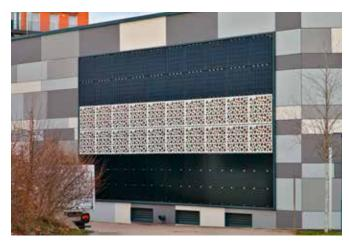
Fig. 3 - Demonstration BIPV façade at Fraunhofer ISE, Freiburg with CIGS (bottom), OPV (middle) and Silicon modules (top) (Photo: © FhG ISE).
