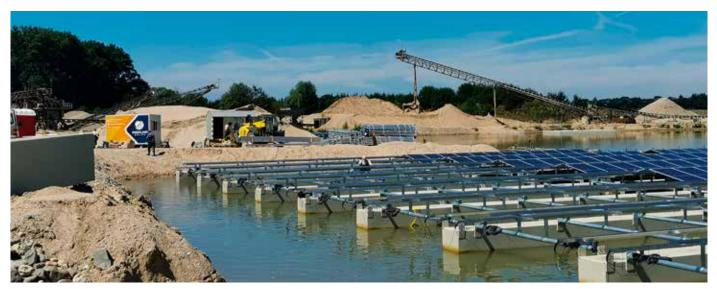
Fig. 6 - 750 kW floating PV on a dredging lake of a gravel pit (Photo: © Energieagentur.NRW / Rheinland Solar).
