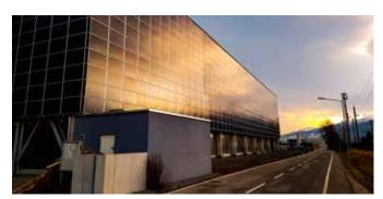
Fig. 2 - M Preis Supermarket's deep-freeze warehouse, Innsbruck, Austria. Winner of the 2<sup>nd</sup> Austrian Award for building integrated PV for their complete energy concept including hydrogen (Photo: © ATB-Becker, Tyrol).
