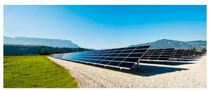
Fig. 1 - A multi-technology photovoltaic test facility for the detailed performance evaluation of different module technologies and mounting systems was set up by EURAC research in cooperation with Airport of Bolzano Dolomiti (ABD). It is operating since 2010 (Photo: EURAC /Othmar Seehauser).
