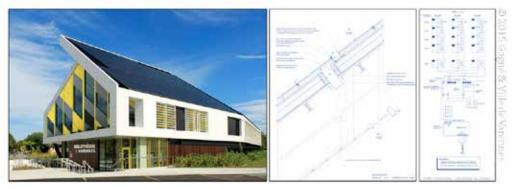
Fig. 2 - One of the selected BIPV projects analysed for the guidebook in preparation: BIPV roof at Varennes Library, Canada, and corresponding technical CAD drawings.
