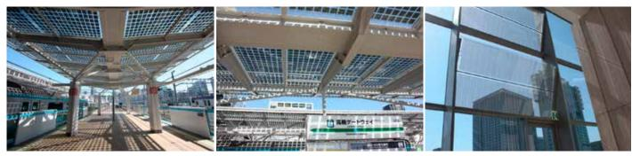
Fig. 1 - Roof and Window Glass-integrated PV System at Station Platform (Takanawa Gateway Station PV System) (Minato Ward, Tokyo). Power generation capacity: 43,8 kW (roof of platform), 1,1 kW (window glass). PV modules: Bifacial single-crystalline silicon PV modules (SUNJOULE® glass-integrated PV modules by AGC).
