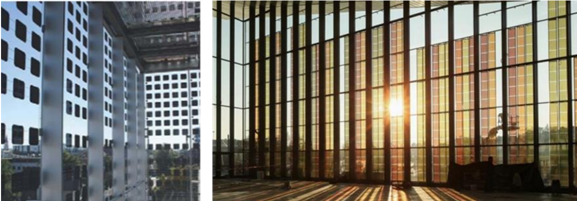
Figure 9. Semi-transparent glazing with c-Si solar cells (left, source: Ertex Solar) and coloured, transparent glazing with dye-sensitised solar cells (right, source: Alain Herzog, Architect: Richter Dahl Rocher)
