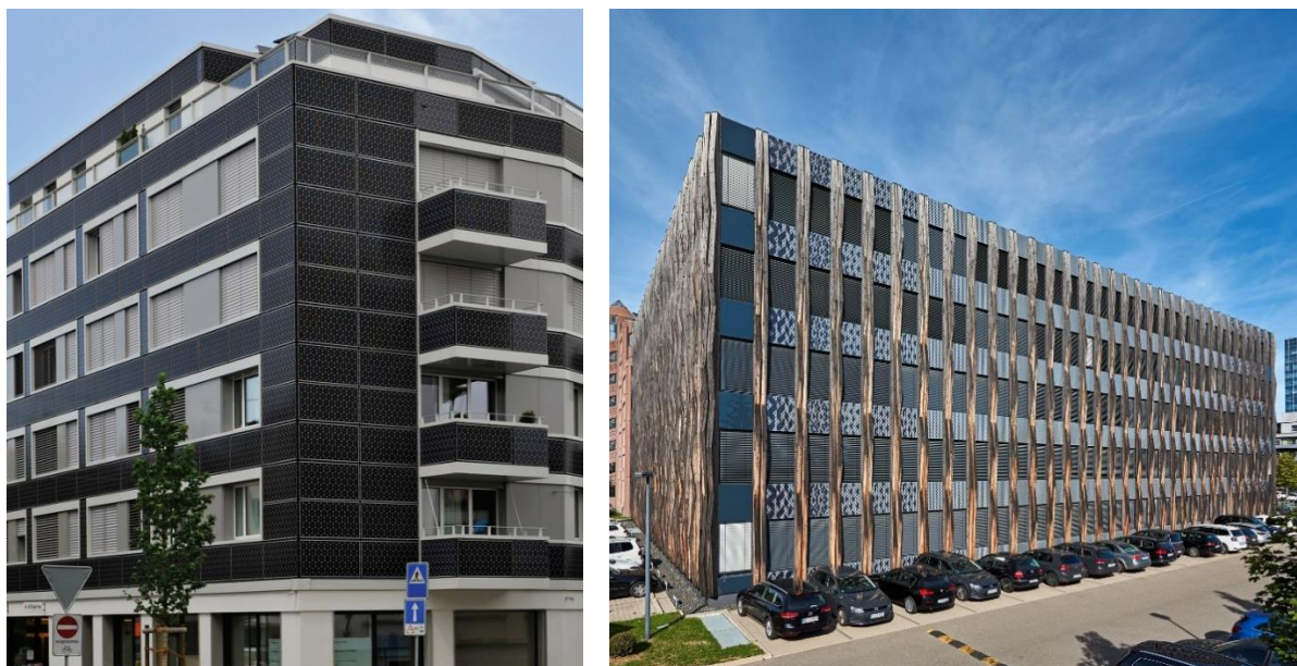
Figure 11. Use of a standard PV architectural language in a multifamily residential in Alleestrass, Romanshorn, Switzerland (left, source: Viridén + Partner) or of a camouflaged appearance in customized PV glazing in the Z3 demonstration building in Stuttgart (right, source: Ed. Züblin AG)
