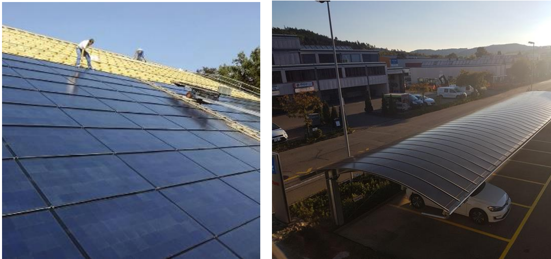
Figure 10. Flat discontinuous rigid roof with regular modules (left, source: Schweizer) and curved carport roof with large flexible modules (right, source: Flisom)
