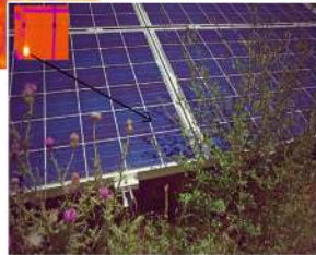
Shading losses (poor vegetation management)
