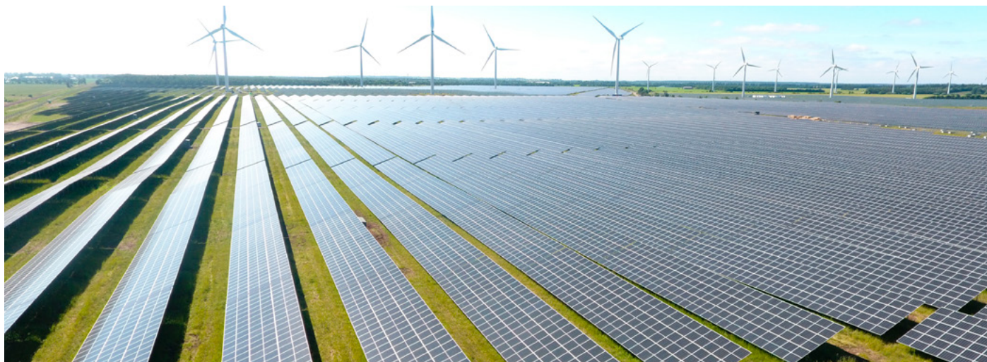
Fig.48 - Better Energy has built the largest solar park in Denmark. The solar park will supply Bestseller, Normal and Nemlig with new green energy. The plant has a capacity of 207 MWp installed.
