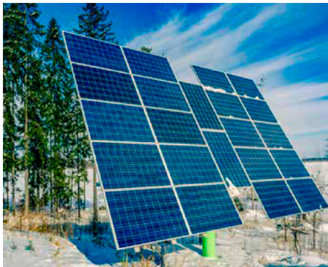
Fig.52 - LUT two-axis tracking solar PV system (Photo: Teemu Leinonen)
