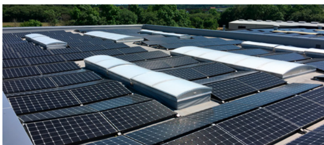
Fig.51 - Haarup Maskinfabrik. The installed 1 MW PV system can supply all the electricity needed in the factory. Batteries with a capacity of 943 kWh improve the self-consumption from the solar plant. For more detailed information see Green transition (haarup.com)
