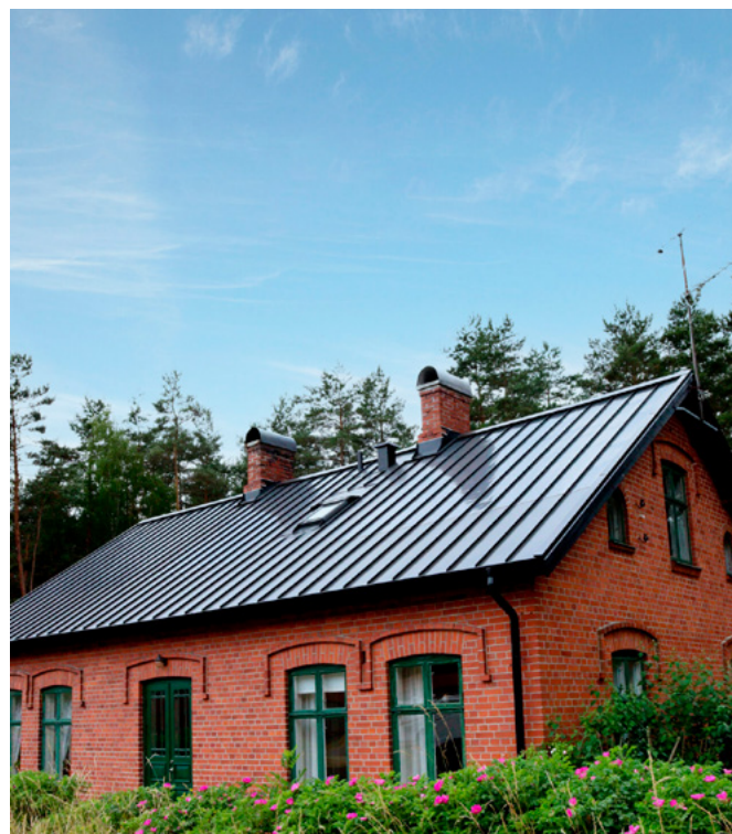
Fig.79 - Folded sheet metal roof with integrated CIGS solar cells, manufactured in Sweden by the company Midsummer. The roof has a PV capacity of 10,7 kW and is located in Österlen. (Photo: © Midsummer).
