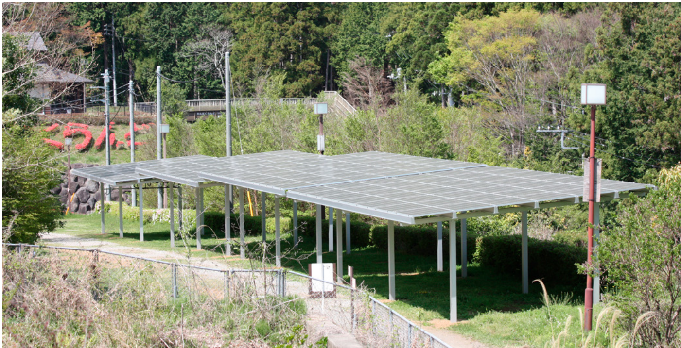
Fig.60 - PV system for regional microgrid at Odawara Kodomo no Mori Park Wanpaku Land in Odawara City, Kanagawa Prefecture, Generation capacity: 50 kW, c-Si PV modules: Kyocera, ©RTS Corporation
