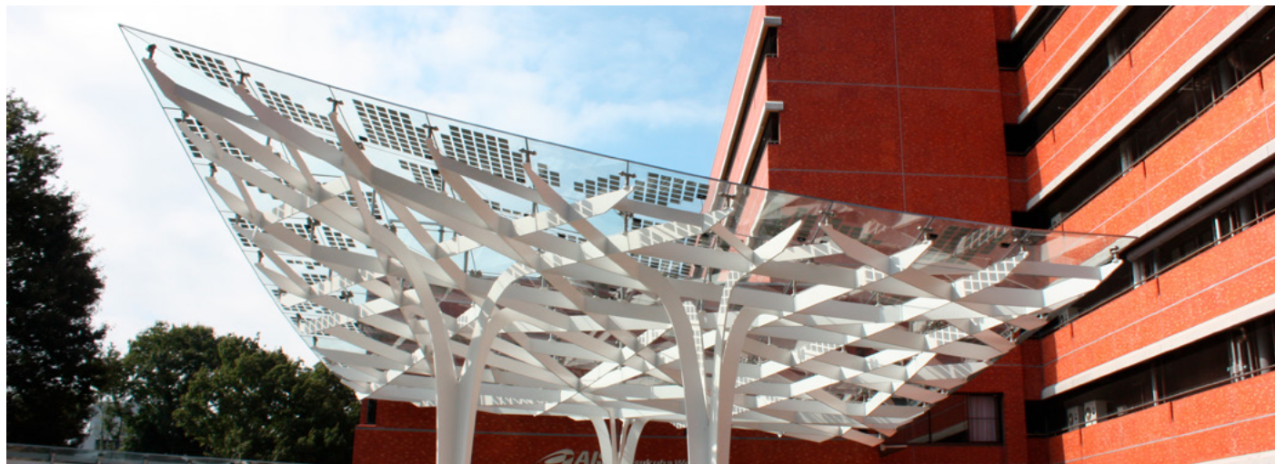
Fig.59 - Canopy type PV system at Global Zero Emission Research Center (GZR), AIST in Tsukuba City, Ibaraki Prefecture, Generation capacity: 6.9 kW, PV glass: Sunjoule® by AGC, ©RTS Corporation
