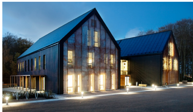
Fig.20 - BIPV roofs for the zero-energy Våla Gård office, Helsingborg (SE), © Skanska Torben Ådahl
