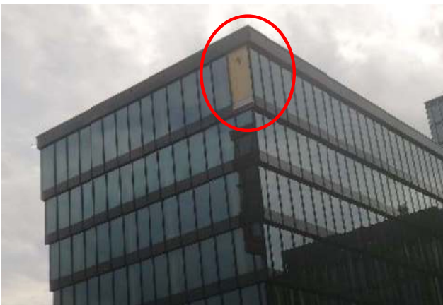
glued glass façade after rupture of the bond
