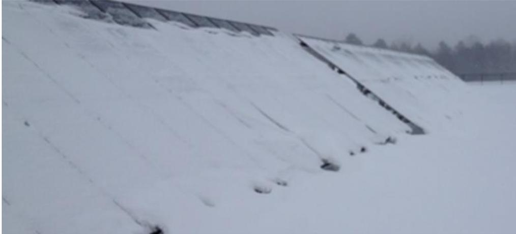
**Figure 58: Insufficient elevation of a PV array can result in snow build-up from the ground that prevents further snow sliding.**
