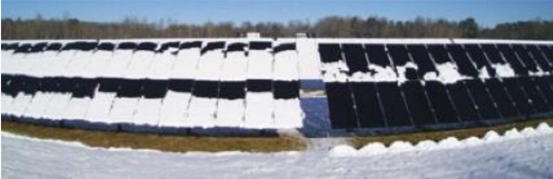
**Figure 53: Framed vs. frameless modules side-by-side PV arrays demonstrate the impact of a module frame on snow shedding. Frameless modules (right) generated 13% more energy in the month of December than the adjacent framed modules. The modules were virtually identical except for the presence or absence of a frame [170].**
