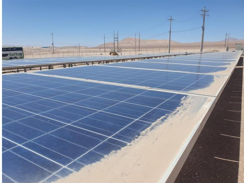
**Figure 16: Soiling pattern demonstrating dominant wind direction.**
