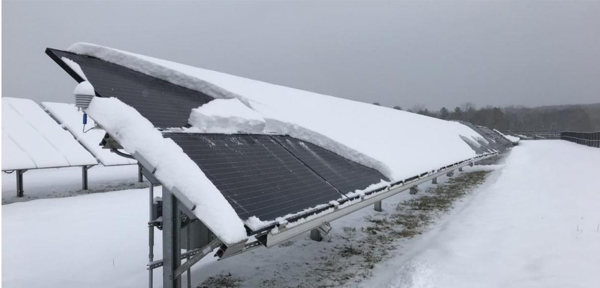
**Figure 52: Uneven snow shedding across PV arrays can make snow depth a challenging indicator of performance.**
