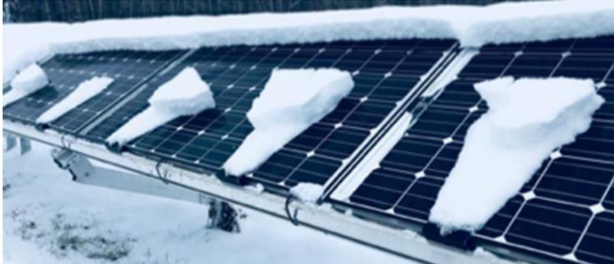
**Figure 57: Module clips.** The photo demonstrates how a module clip can create a physical barrier that prevents snow from sliding from the module surface.
