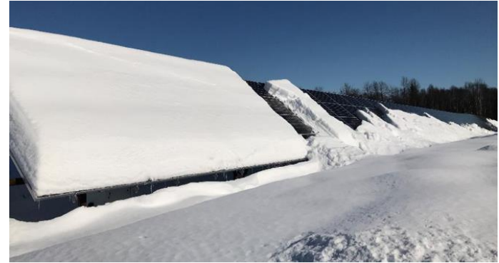
Snow covered array [Alaska, USA]
