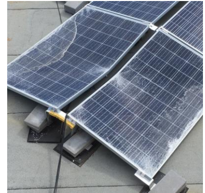
Snow drift on rooftop-PV and broken modules [Piteå, SE]
