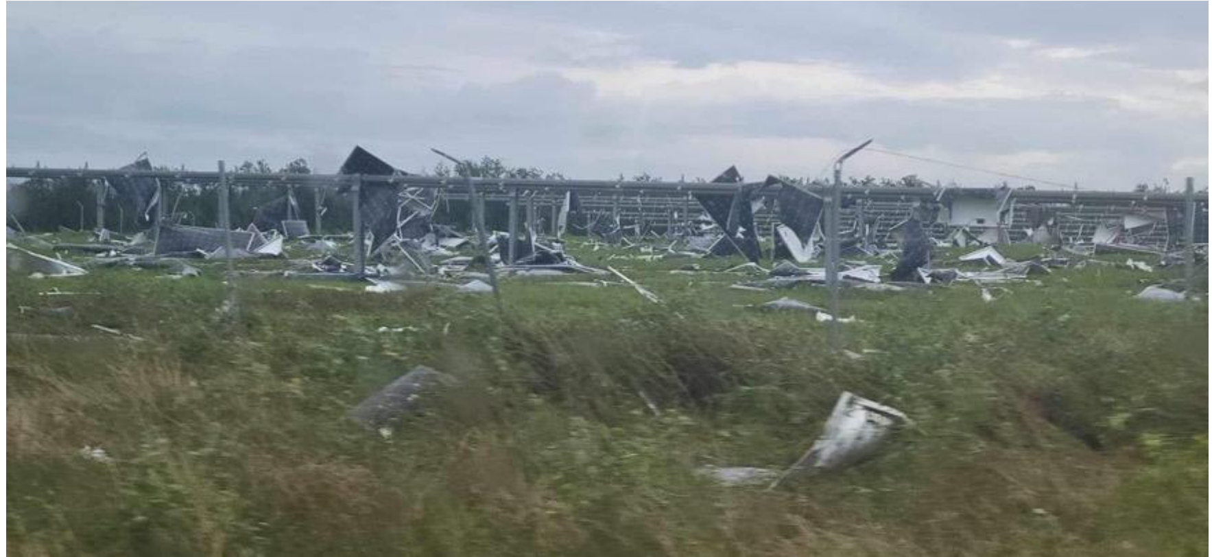
Hurricane Milton, October 2024
