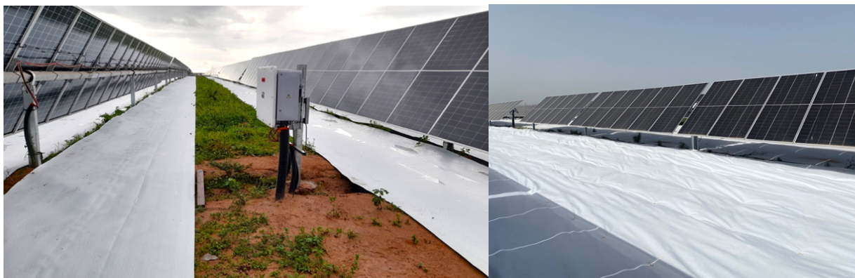
Figure 11 – Two examples for applications of albedo enhancers under bifacial trackers in large-scale PV power plants. Left: large-scale test of Solmax's Geolux albedo sheets (geomembranes) in Brazil (photo: Recurrent Energy), Right: Magnifield albedo enhancers (geotextiles) installed in a multi-MW power plant in Italy.
