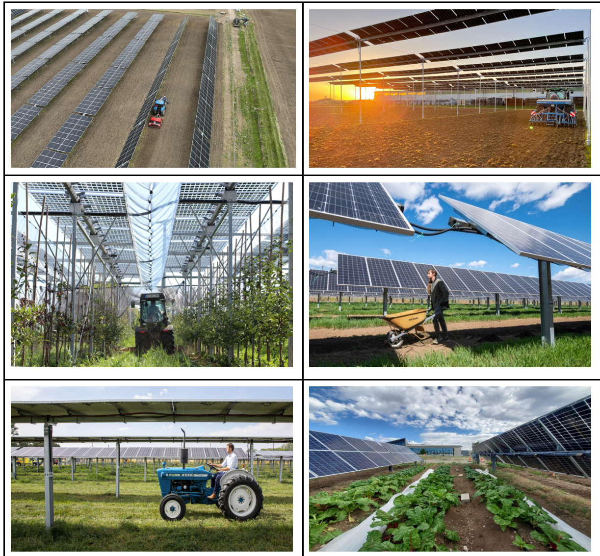
Figure 16 – (top left): Custom 2P tracker angle positioning during interrow crop sowing in Denmark (photo credit: European Energy), (top right): overhead trackers from HyPERFarm European project (photo credit: Fraunhofer ISE) , (center left): overhead semitransparent trackers in apple orchard in Bavendorf, Germany (photo credit: Fraunhofer ISE), (center right and bottom left): Jack's Solar Garden in Longmont, Colorado (Photo credit: NREL), (bottom right) NREL agrivoltaic testbed in Golden CO, U.S.A.
