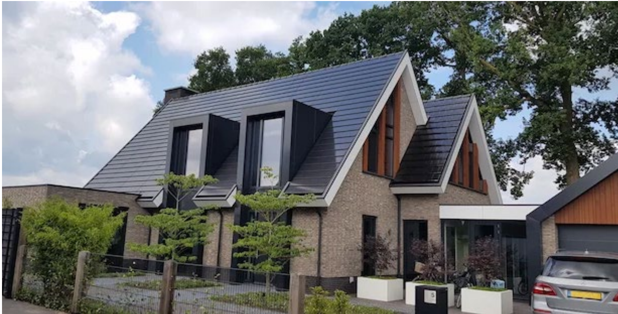
Figure 2. In-Roof solar panels, RVO database
