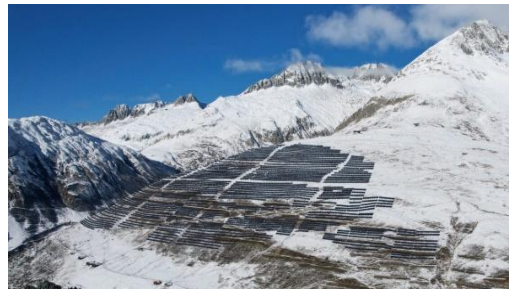
Sedrun Solar (2029 m.a.s.l.), 19.3 MW system under construction
