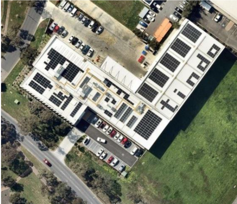
Figure 13 - Tindo Manufacturing Line rooftop. Image provided by Tindo Solar.
