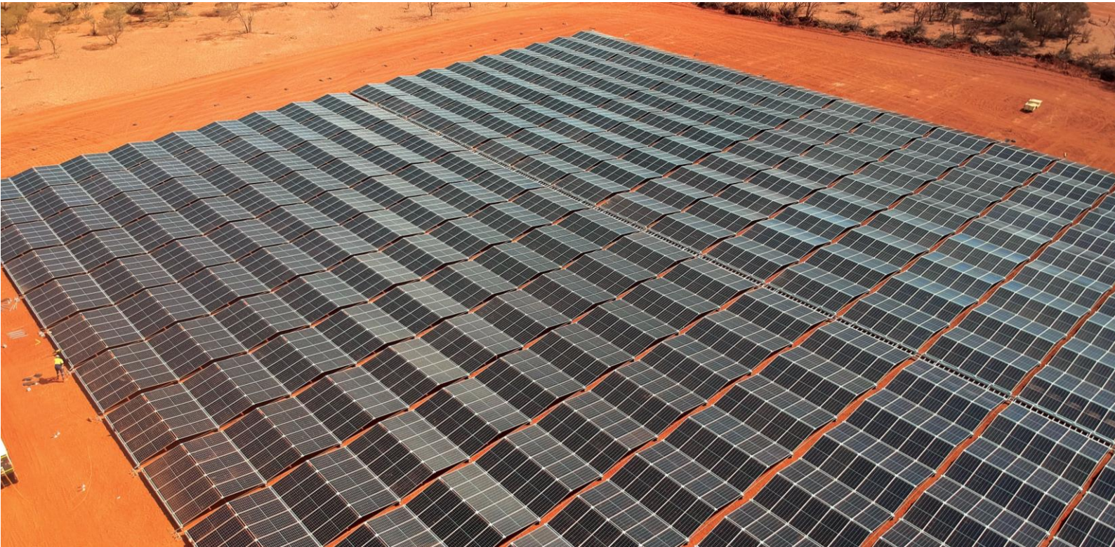
Figure 6 - 30 MW King of the Hills Solar Farm. Image provided by 5B Pty Ltd
