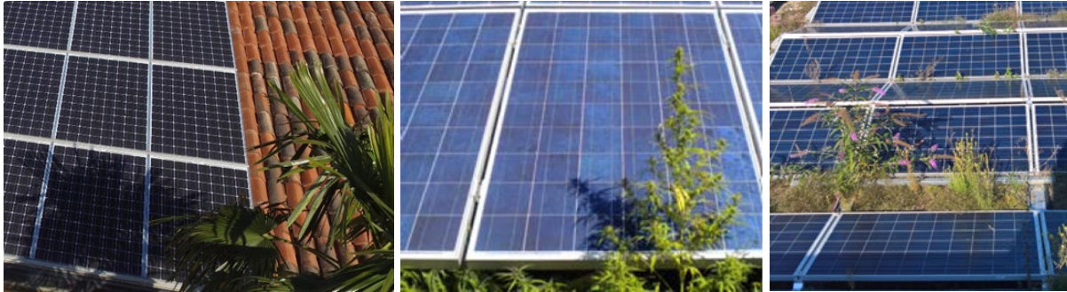
Figure 15: Shading due to (a) trees and (b) vegetation. Images from [34] and [31], respectively.
