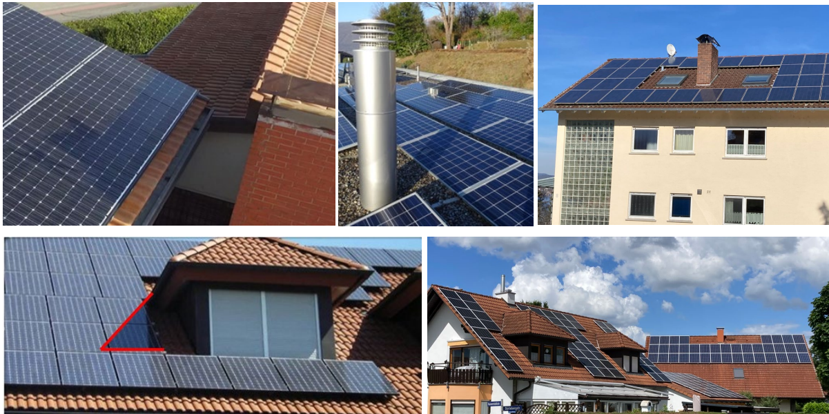
Figure 14: Shading due to (a) another building, (b) the chimney and (c) the dormer [19]. Images from [34].
