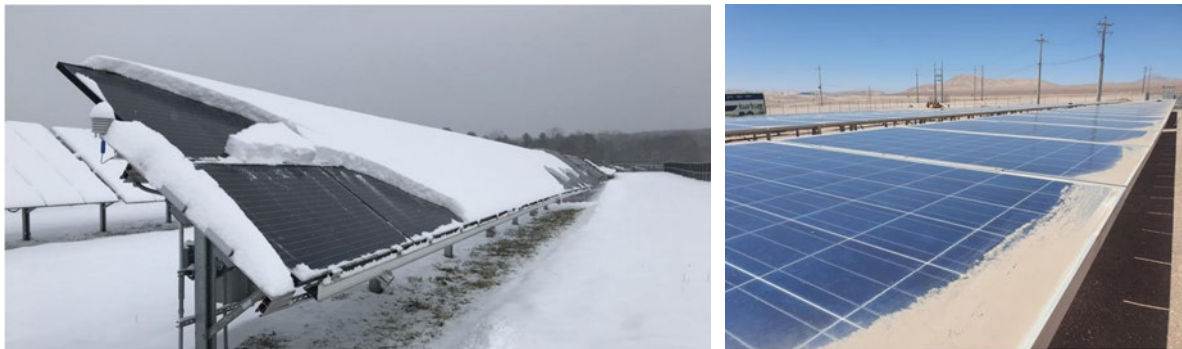
Figure 12: Shading due to (a) snow and (b) soiling. Images from [32].
