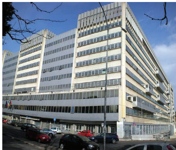
Figure 5.102 Pedestrian view of Palazzo Argonauta before renovation. Credits: DiARC.
