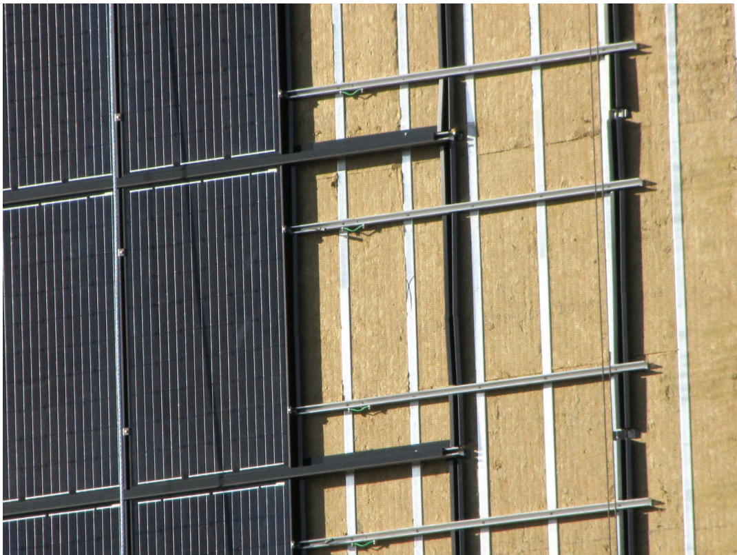
Figure 5.69 Detail of the BIPV rainscreen at Jeanne & Peter Loughheed Performing Arts Centre. Credits: Gordon Howell, HME.
