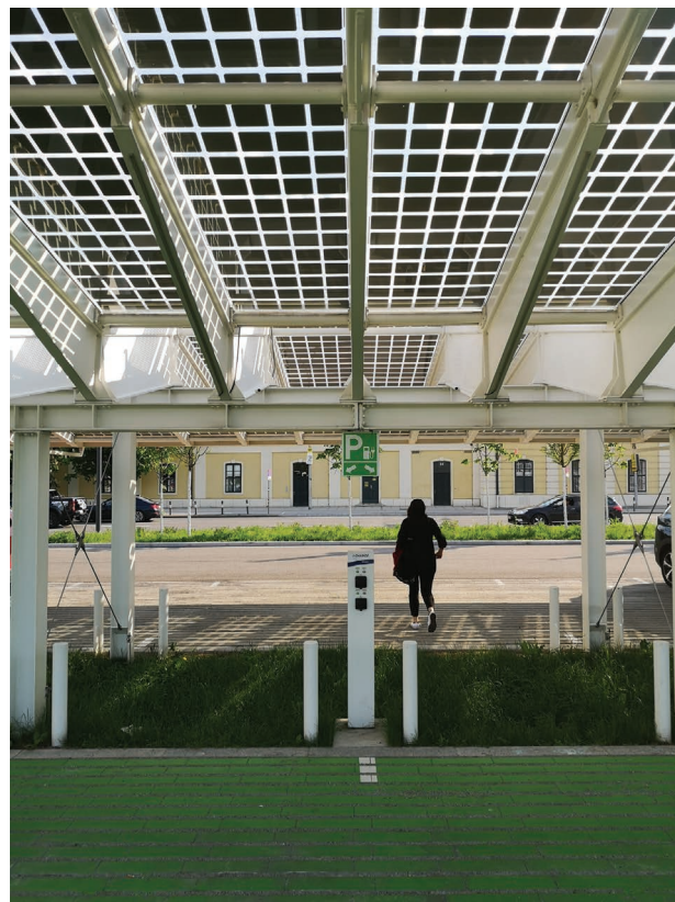
Figure 5.137 Close-up view of the BIPV car canopy at the arrival centre in Schönbrunn. Credits: Francesco Frontini, SUPSI.
