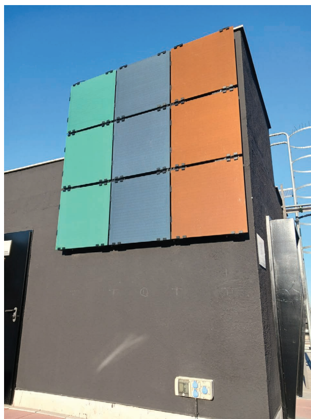
Figure 2.1 Coloured demonstration façade at CIEMAT, Spain. In this example, green and terracotta BIPV modules reduce the efficiency by 4% and 15%, respectively, when compared to the anthracite colour. Ref: RINGS-BIPV project, 2023. Source: N. Martín-Chivelet, CIEMAT.
