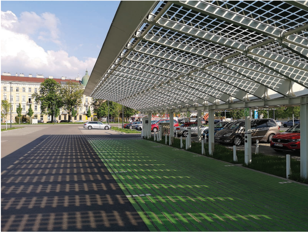
Figure 5.136 BIPV car canopy at the arrival centre in Schönbrunn. Credits: Francesco Frontini, SUPSI.
