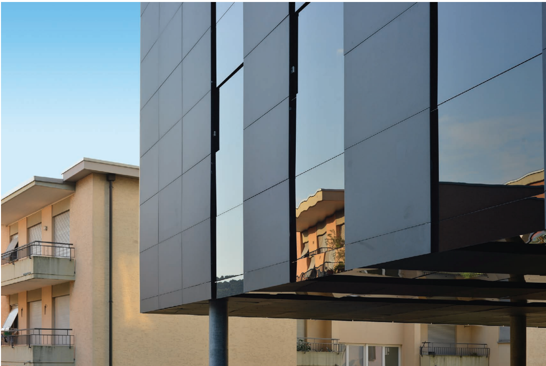
Figure 5.80 Detail of the DeltaROSSO BIPV rainscreen. Credits: Isa Zanetti, SUPSI.
