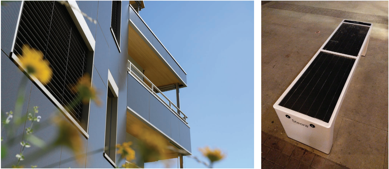
Figure 3.16 From balustrades to solar benches, BIPV can take several forms within the built environment. Photos: courtesy of Isa Zanetti (left) and Costa Kapsis (right).
