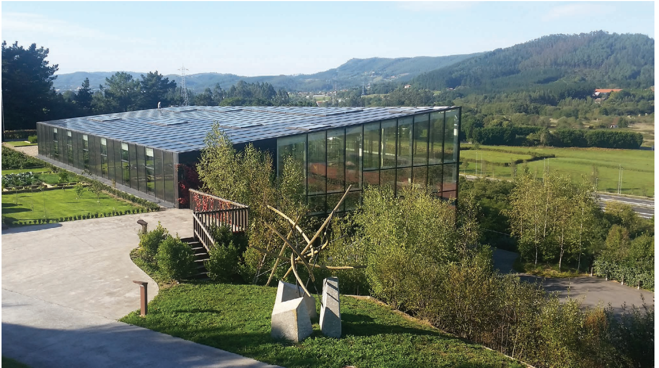
Figure 5.49 General view of Azurmendi Restaurant showing the BIPV façade and skylight. Credits: Onyx Solar.
