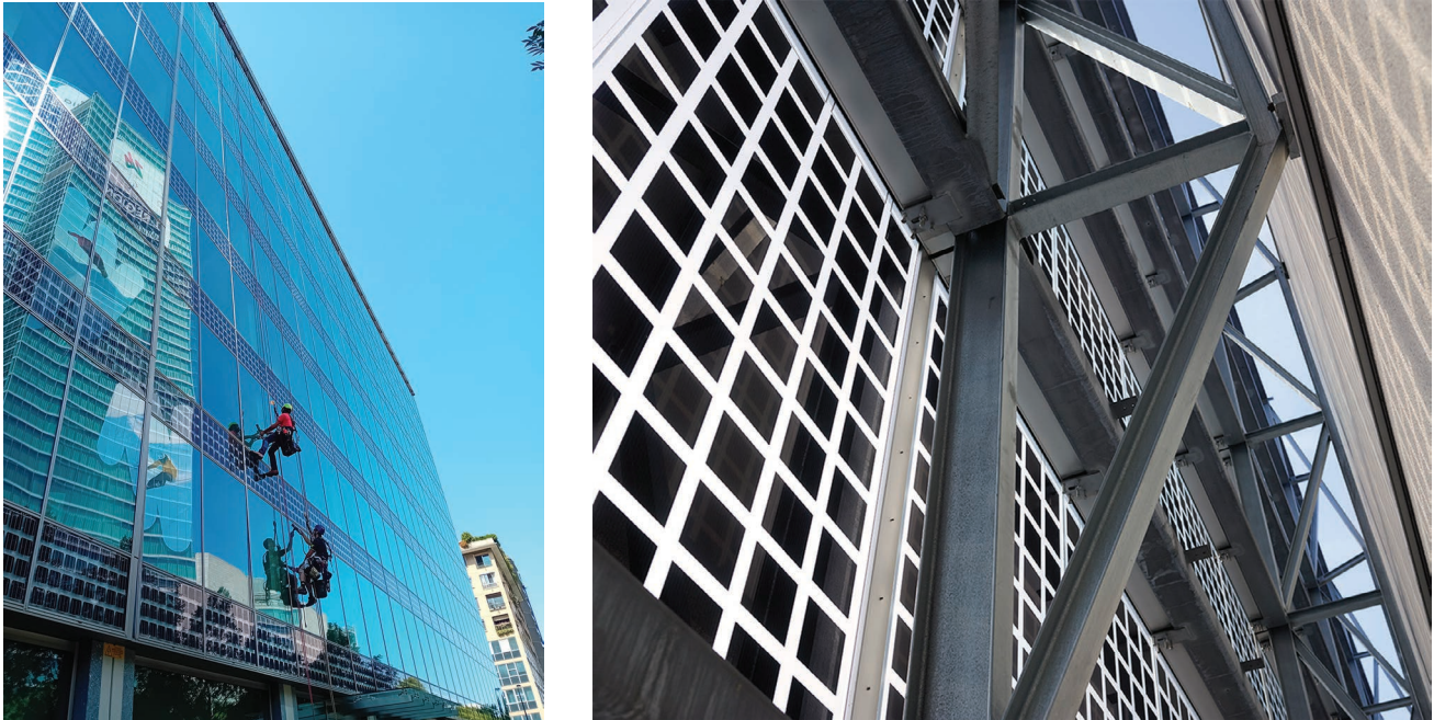
Figure 3.12 Double-skin façades featured in a new office building in Milan, Italy, and the renovated CSEM building in Neuchâtel, Switzerland. Photos: courtesy of P. Bonomo, SUPSI.
