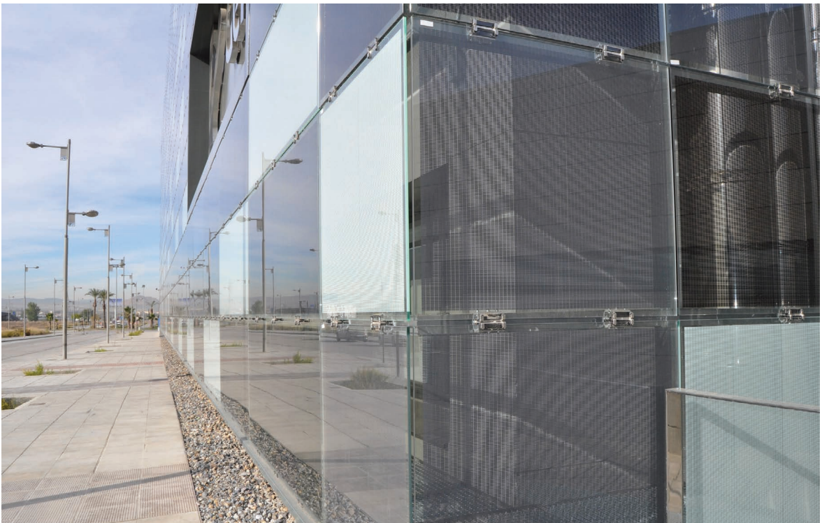
Figure 5.97 Detail of the BIPV double skin façade of the Genyo Research facility. Credits: Onyx Solar.
