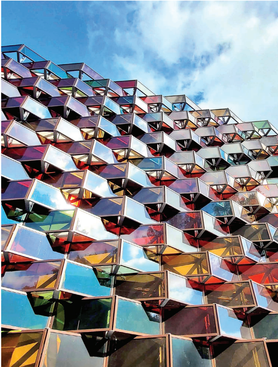
Figure 5.125 Coloured transparent BIPV shading at Gothenburg Garage. Credits: Soltech Energy Sweden.
