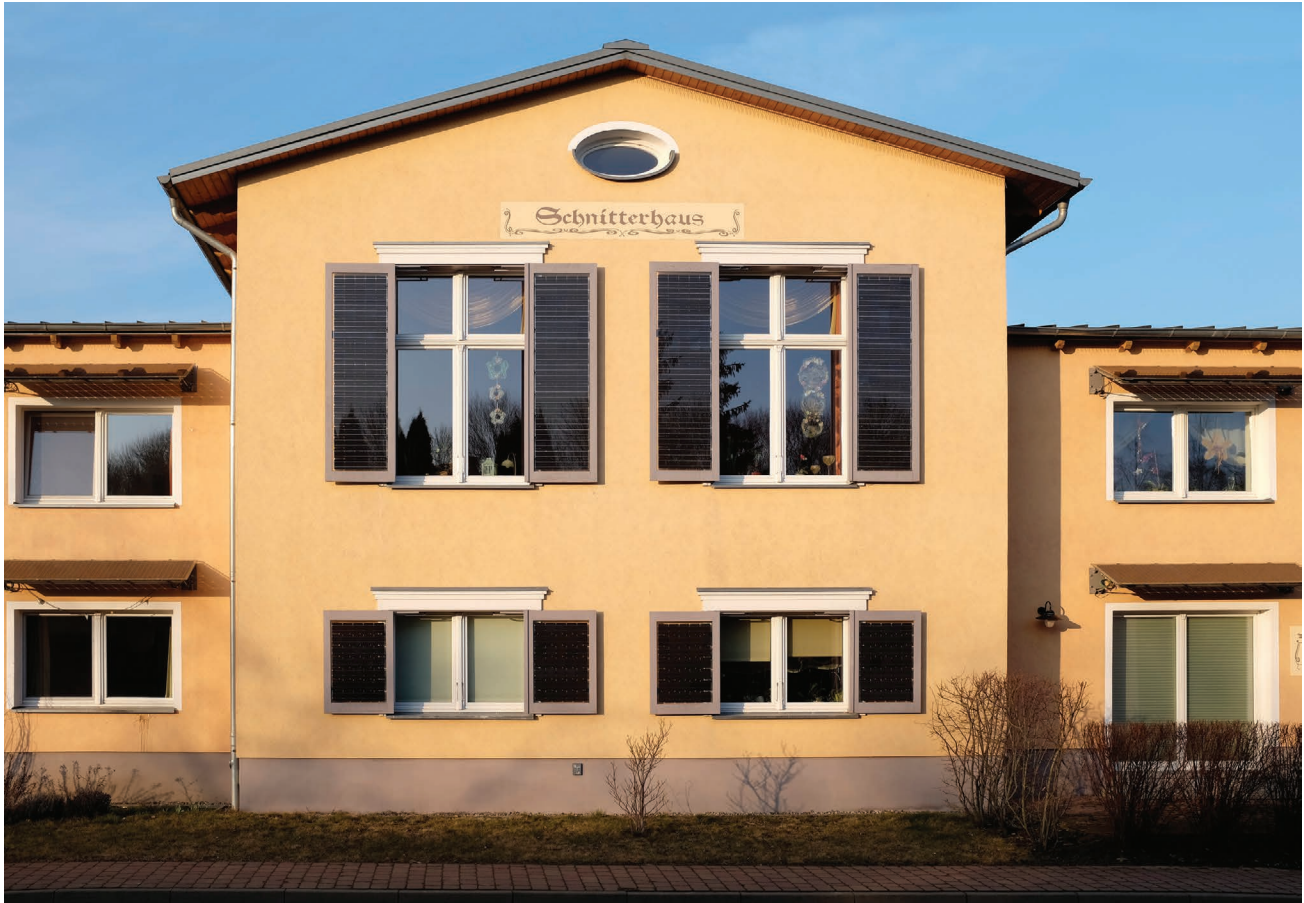
Figure 3.15 Residential building in Nechlin, Germany, with “Solar Window Shutters” designed and patented by Astrid Schneider. Photo: Astrid Schneider, Solar Architecture, Berlin.
