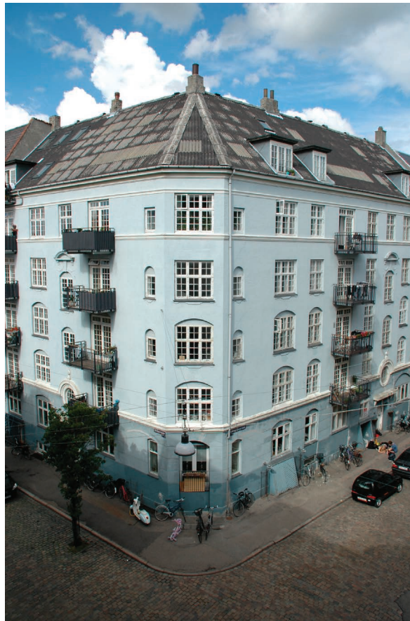
Figure 5.32 Andreas Bjørns St.1 before renovation. Credits: Solar City Denmark.
