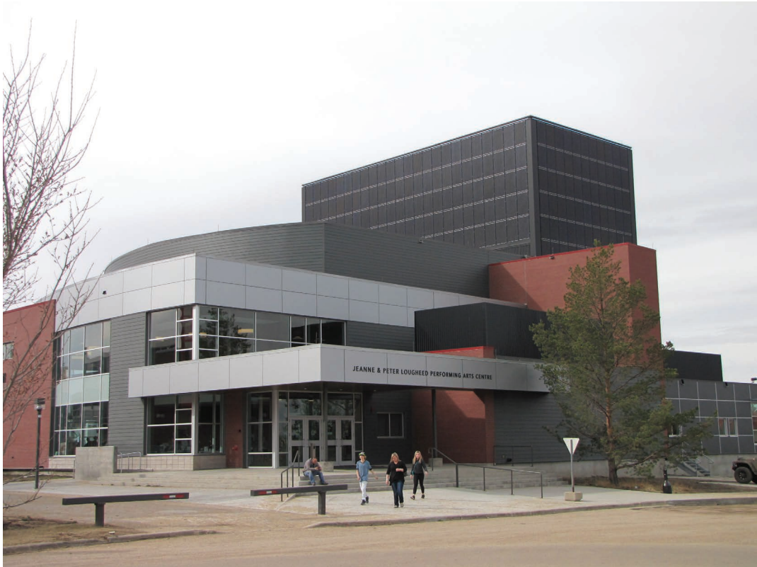
Figure 5.68 Pedestrian view of Jeanne & Peter Loughheed Performing Arts Centre. Credits: Gordon Howell, HME.
