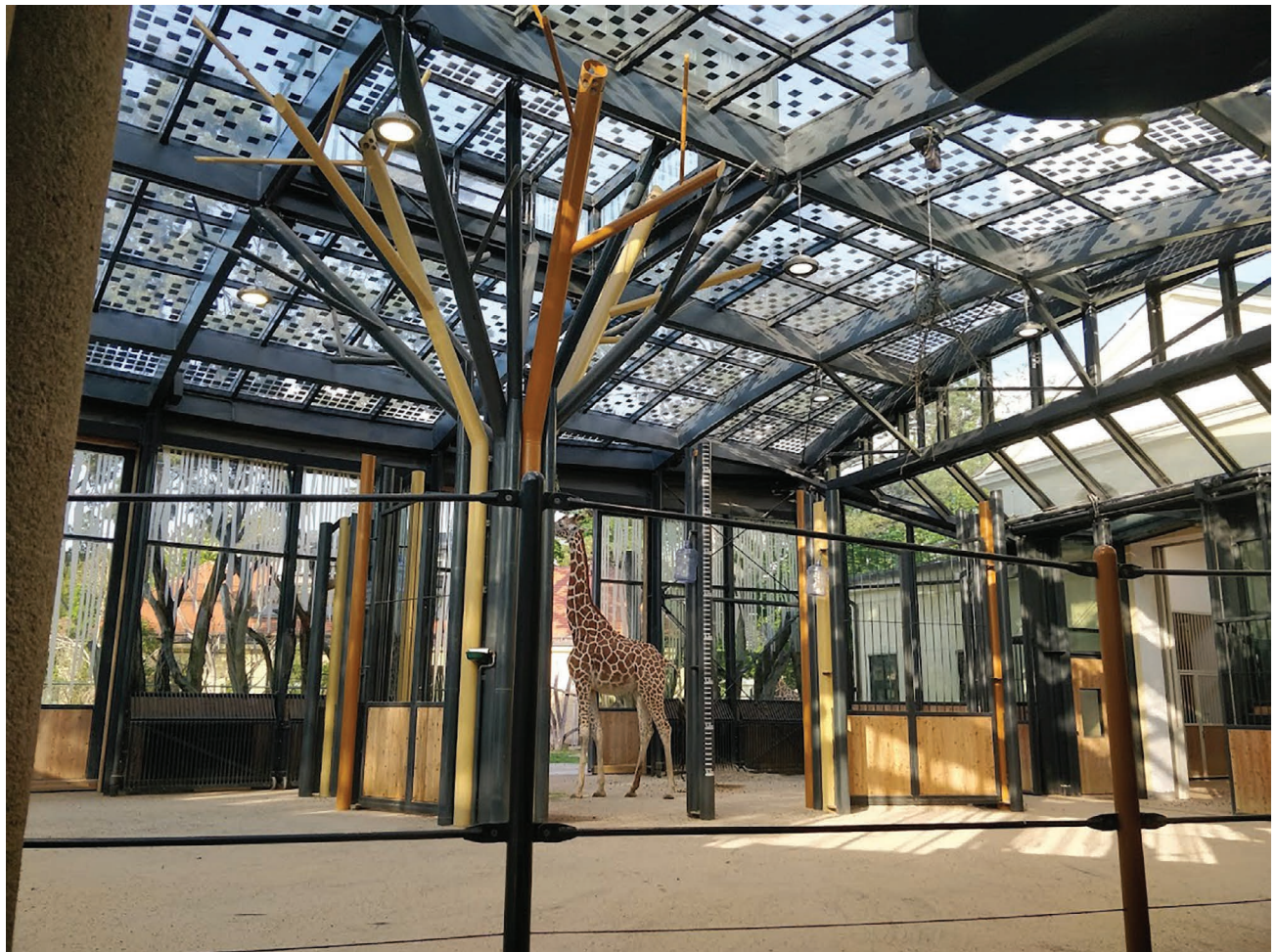
Figure 3.5 BIPV skylight at the Schönbrunn Zoo, in Vienna, using customised solar cell patterns. Photo: Costa Kapsis.
