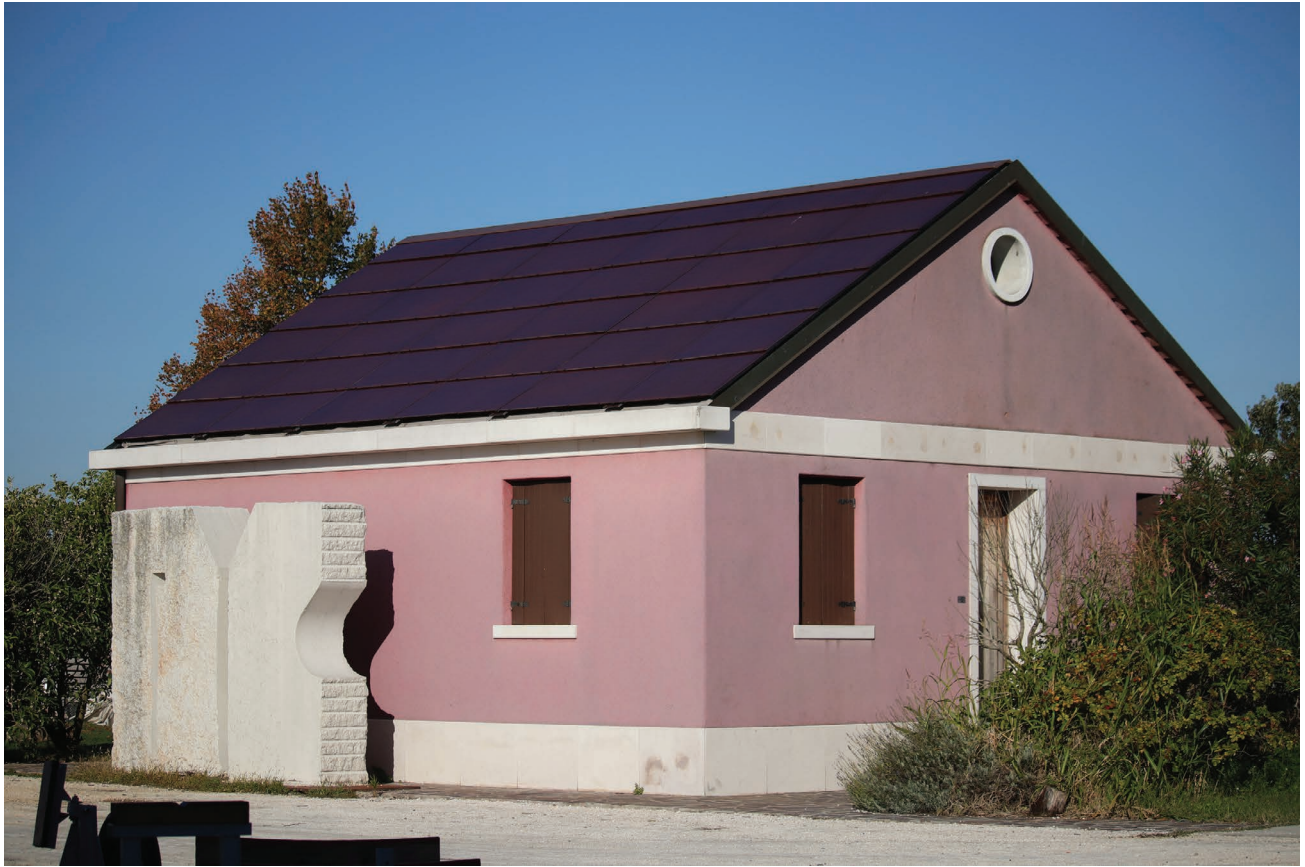
Figure 5.37 BIPV roof in a heritage building at the Urban Park in Certosa Island. Credits: GruppoSTG.
