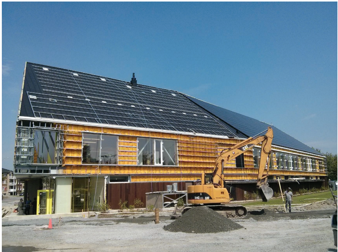
Figure 5.5 Varenes library under construction. Credits: Jose Candanedo.
