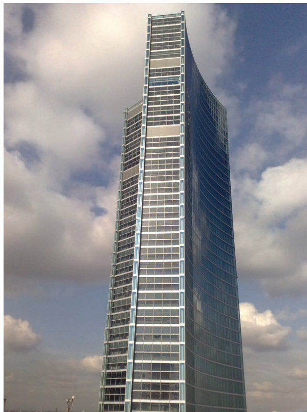
Figure 5.119 BIPV unitised curtain wall façade at Palazzo Lombardia. Credits: DiARC.
