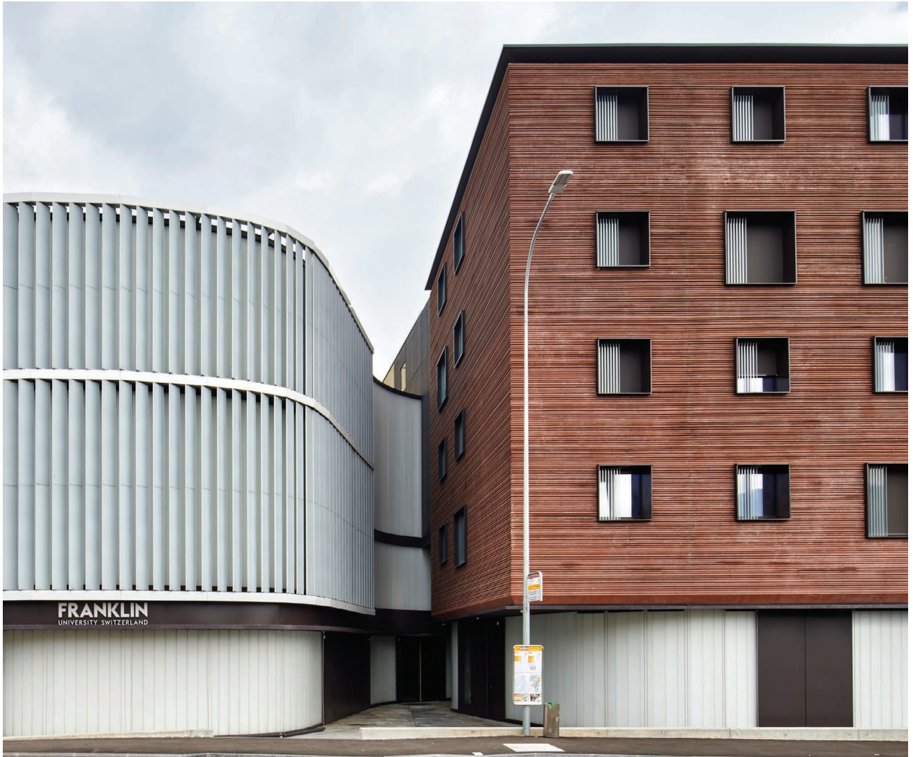
Figure 5.130 Pedestrian view of Franklin University Student Residence. Credits: Franklin University.
