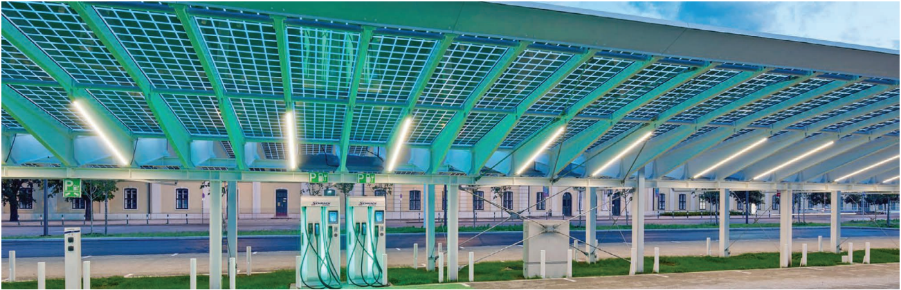
Figure 5.138 Night view of the BIPV car canopy at Schönbrunn. Credits: Ertex solar.
