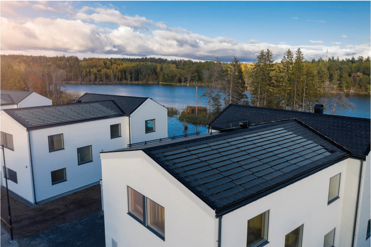
Figure 5.28 Close-up view of the Glasberga BIPV roofs. Credits: Soltech Energy Sweden.
