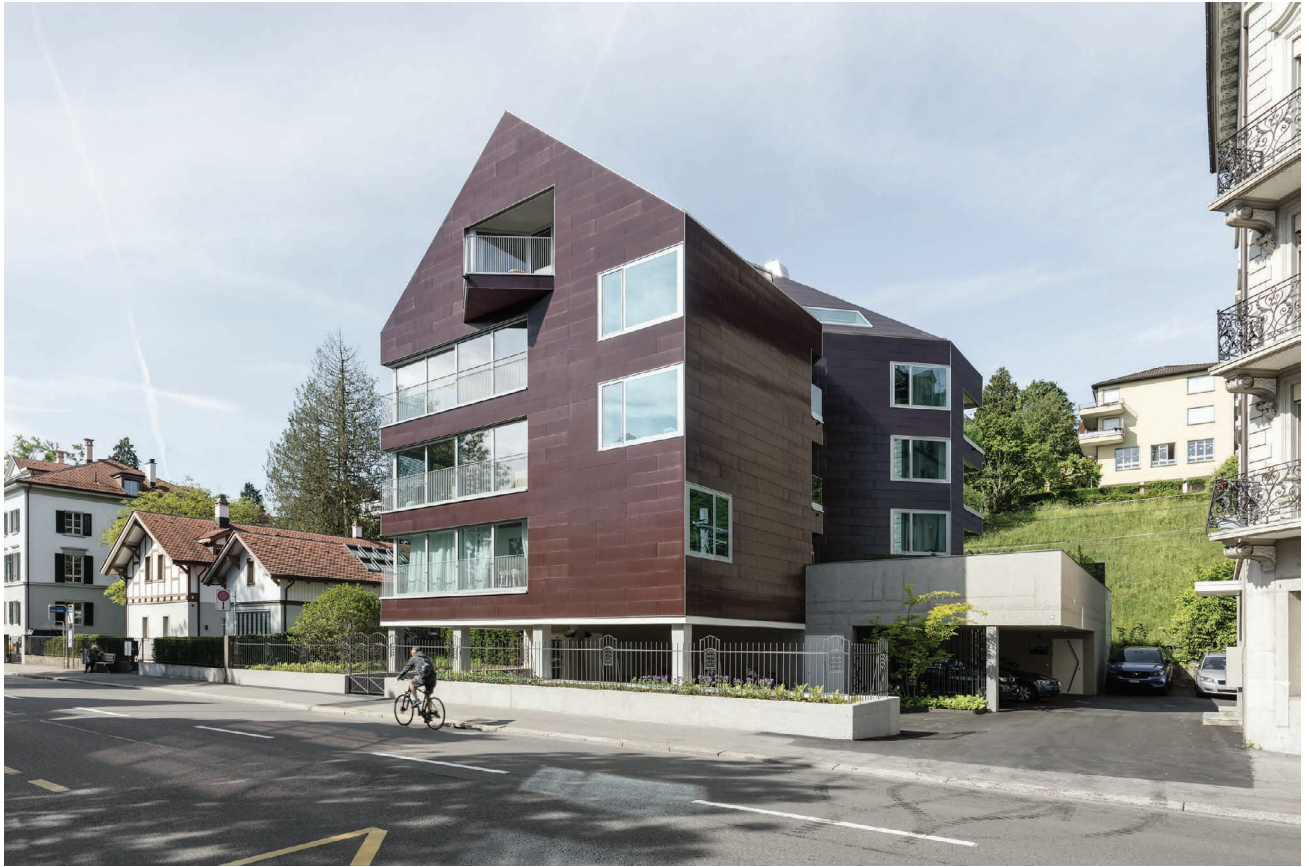
Figure 5.21 Front view of the Solaris 416 building. Credits: Isa Zanetti, SUPSI.
