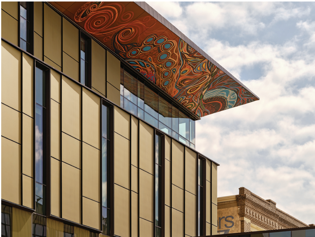
Figure 5.86 BIPV rainscreen detail of Manitou a bi Bii Daziigae building. Credits: Diamond Schmitt Architects.
