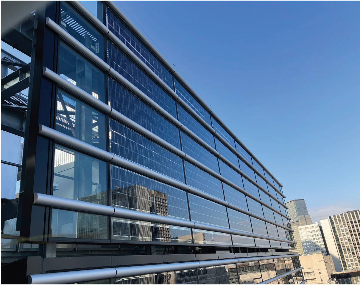
Figure 5.109 Detail of the Yanmar BIPV curtain wall. Credits: Yanmar.
