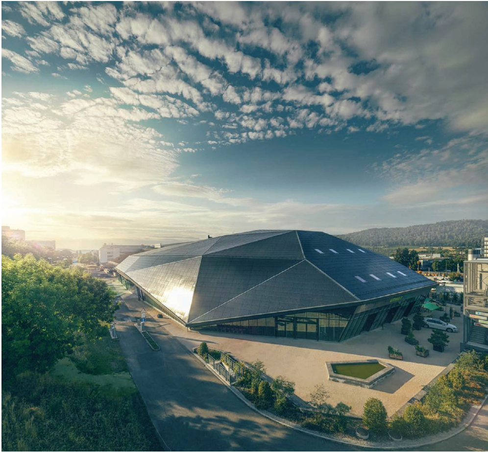
Figure 5.10 Panoramic view of Umwelt Arena. Credits: Isa Zanetti, SUPSI.
