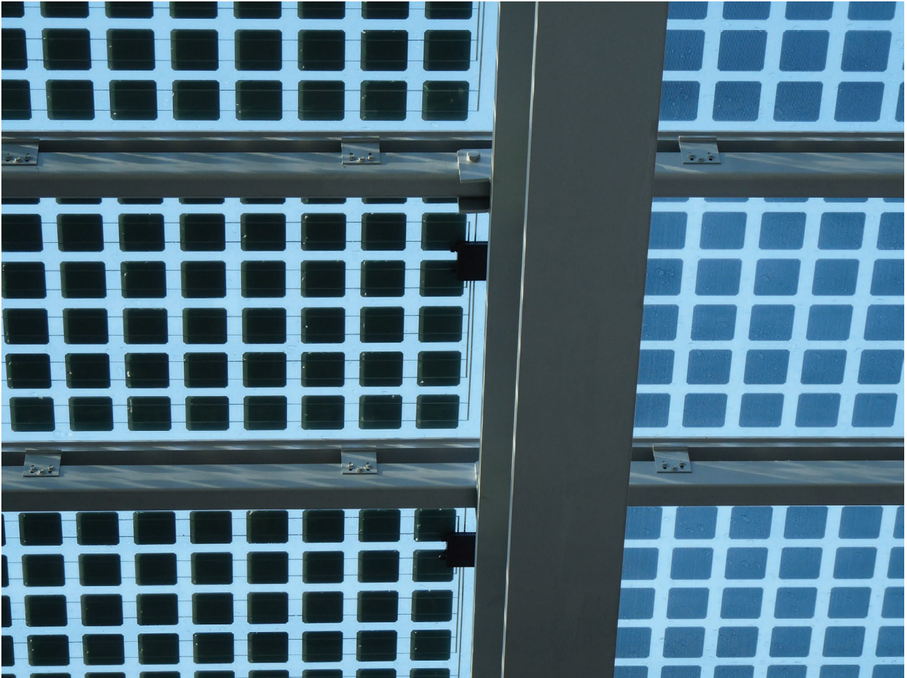
Figure 5.63 Detail of the BIPV skylight and dummy modules. Credits: Francesco Frontini, SUPSI.
