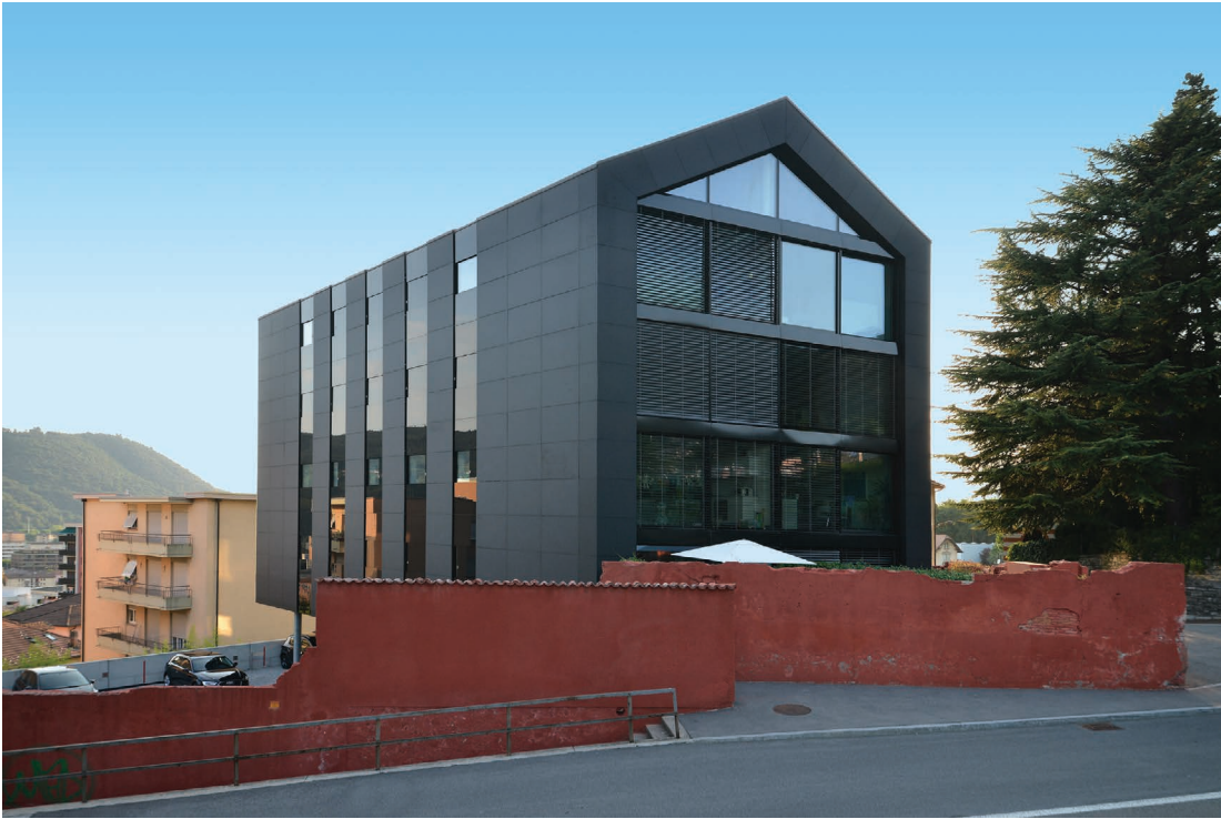
Figure 5.79 Pedestrian view of DeltaROSSO building. Credits: Isa Zanetti, SUPSI.
