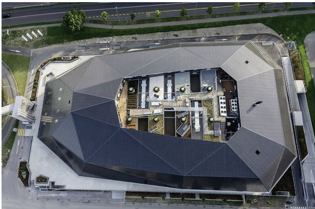
Figure 5.11 Eagle-eye view of Umwelt Arena. Credits: Isa Zanetti, SUPSI.
