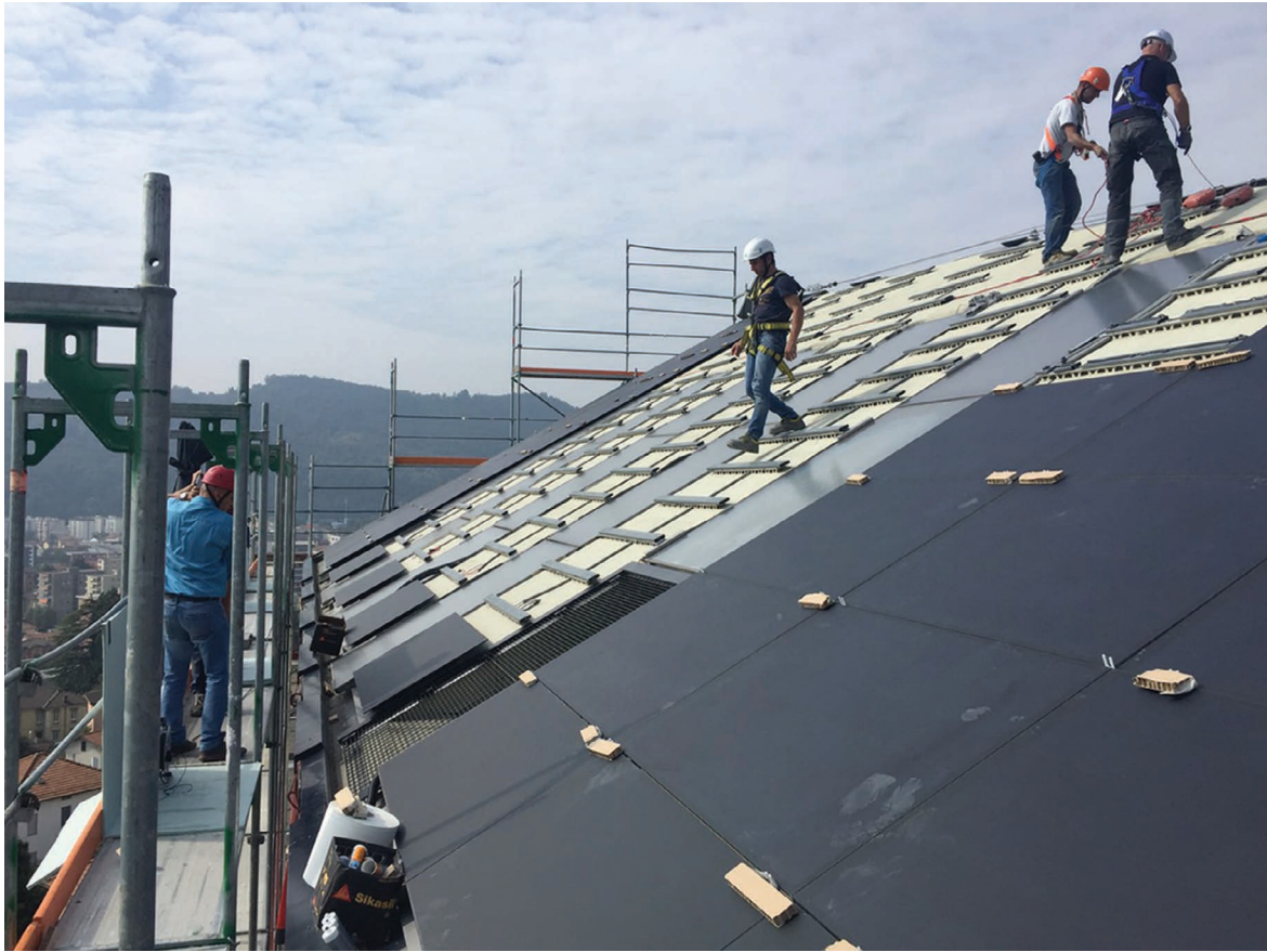
Figure 5.81 DeltaROSSO BIPV ventilated roof under construction. Credits: Isa Zanetti, SUPSI.
