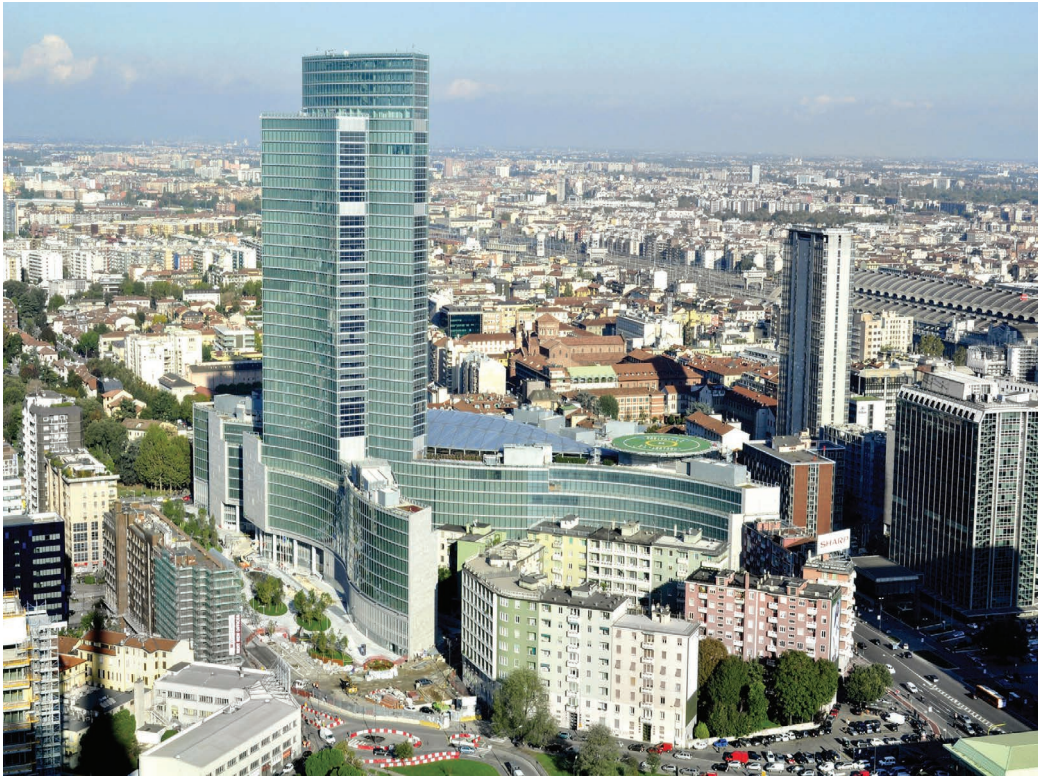
Figure 5.118 Eagle-eye view of the Palazzo Lombardia complex. Credits: Caputo & Partners.
