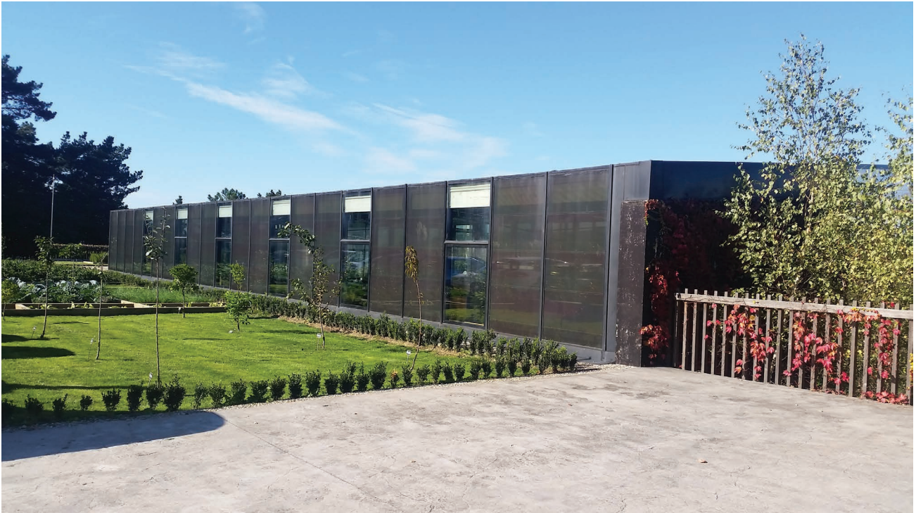
Figure 5.51 Semitransparent curtain wall at the Azurmendi Restaurant. Credits: Onyx Solar.
