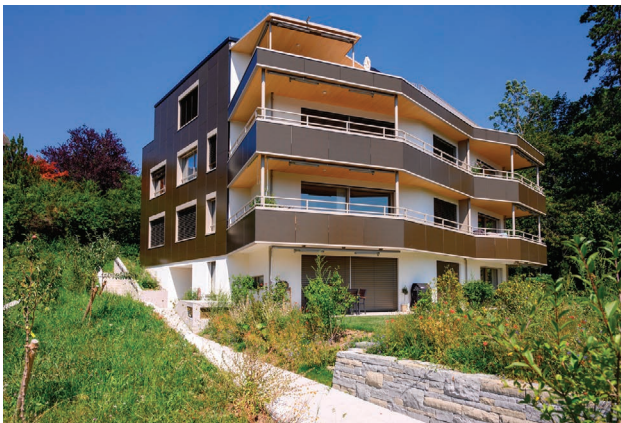
Figure 3.11 Rainscreen cladding with coloured modules in a multi-family house in Zurich, Switzerland, designed by Kämpfen Zinke + Partner AG. Photos: courtesy of I. Zanetti, SUPSI.
