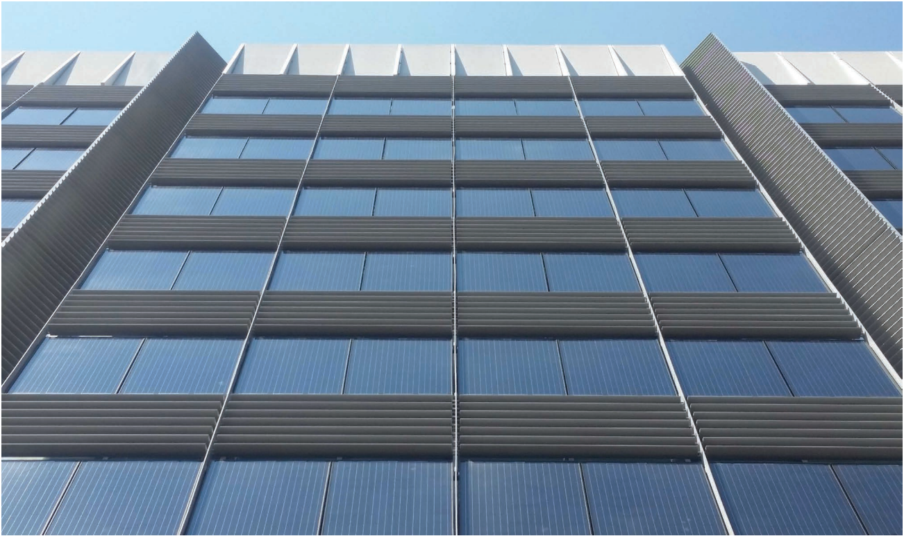
Figure 5.103 Close-up of the Palazzo Argonauta BIPV rainscreen. Credits: DiARC.
