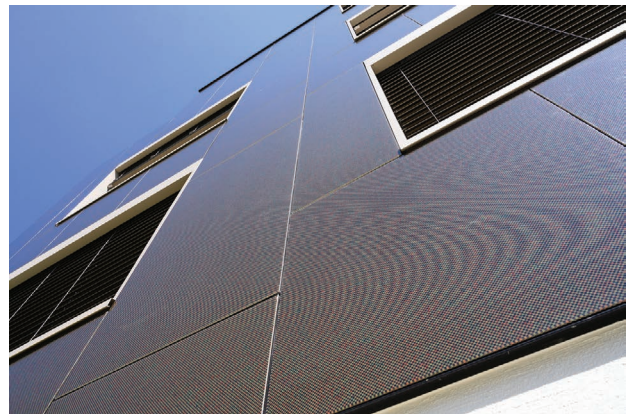
Figure 3.11 Rainscreen cladding with coloured modules in a multi-family house in Zurich, Switzerland, designed by Kämpfen Zinke + Partner AG. Photos: courtesy of I. Zanetti, SUPSI.
