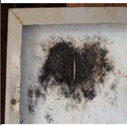
Burn mark at the backsheet with cracked backsheet [Sinclair17].
