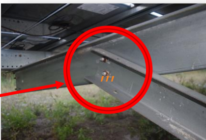
Rails insufficient for load
