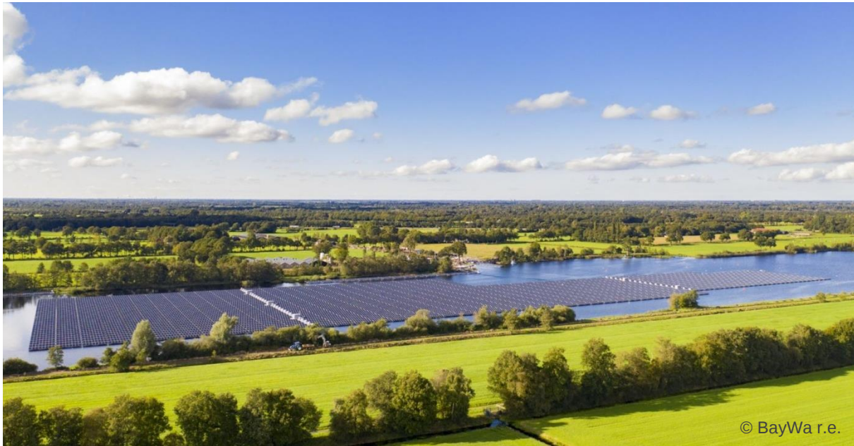
Figure 7. FPV power plant with ZIM Float technology installed in 2021 with a capacity of 13.7 MW at Lippe Gabrielsplas in the Netherlands.
