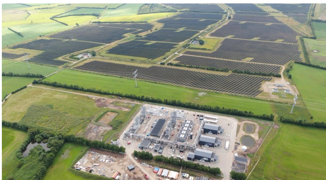
Photo 8: European Energy and Mitsui & Co.s's PtX plant in Kassø with solar park (304 MWp), electrolyser (52 MW) and e-methanol facility (32 000 tonnes per year) co-located in the Aabenraa municipality, Denmark.
