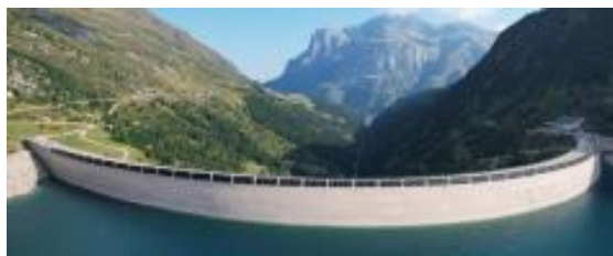
Photo 35: Alpine PV system (343 kW) at the Lago di Lei dam (Source: ©REECH AG, ewz 2022). The findings from the first years of operation with such systems are positive: no critical operational disruptions have occurred and the share of winter solar electricity is high.
