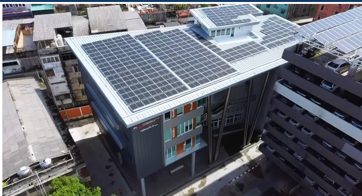
Photo 36: Thailand's largest net-zero energy government building (100 kWp solar PV installed capacity) located at Department of Alternative Energy Development and Efficiency, Bangkok.
