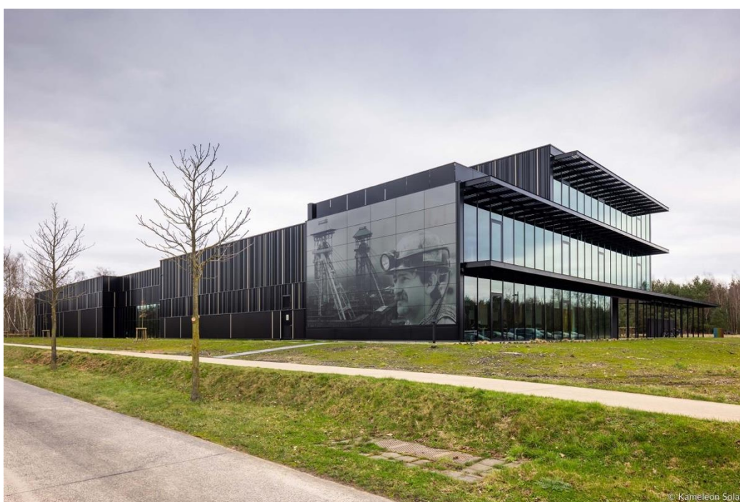
Photo 5: 2024 BIPV Award winning BIPV solar façade from Kameleon Solar and Soltech located in the new Soltech factory in Genk.
