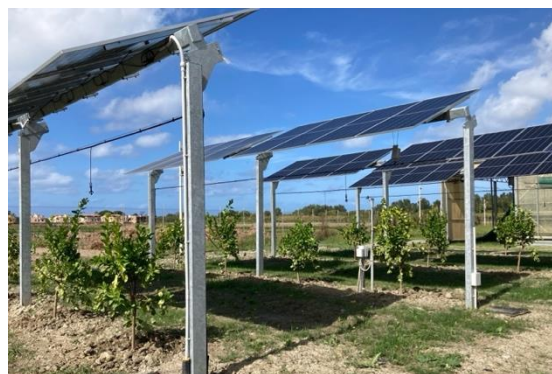
Photo 19: Agrivoltaic demonstrator (fixed system) with lemon trees, in Scalea, realised by ENEA in collaboration with EF Solare Italia, Le Grenhouse and SET Energie. Image: ENEA.
