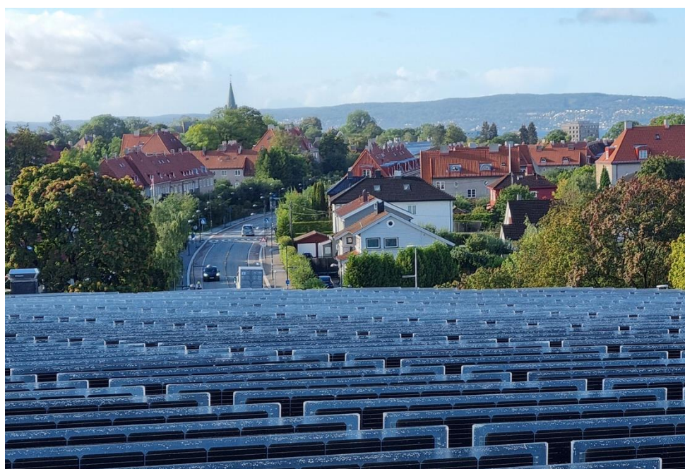
Photo 27: Vertical PV is a good match for high latitudes. Over Easy Solar system on Ullevål Stadion, the Norwegian national football arena. Photo: Jarand Hole.
