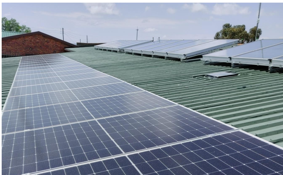
Photo 30: The Solar Photovoltaic – Solar Thermal tandem installation implemented through SOLTRAIN in Bronk-horstspruit, South Africa.
