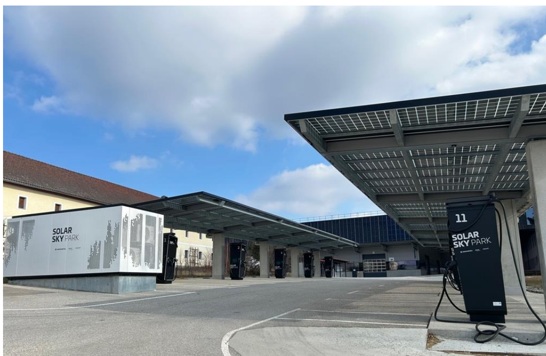
Photo 4: SOLARSKYPARK fast-charging park for e-mobility with neoom outdoor battery storage and solar carport.
