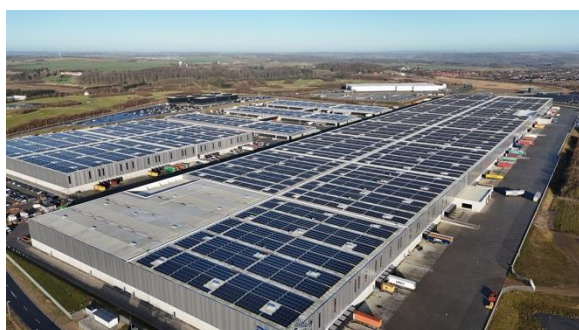
Photo 9: 35 MWp east/west orientated roof top system installed on a DSV building in Horsens. The system is installed by SolarFuture.
