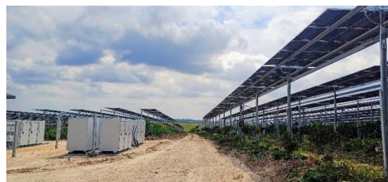
Photo 17: Hybrid PV-plus-Storage Installation in a Solar Farm.
