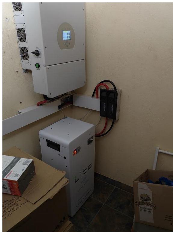
Photo 31: The Solar Photovoltaic Inverter and Battery Backup installation implemented through SOLTRAIN in Bronkhorstspuit, South Africa.
