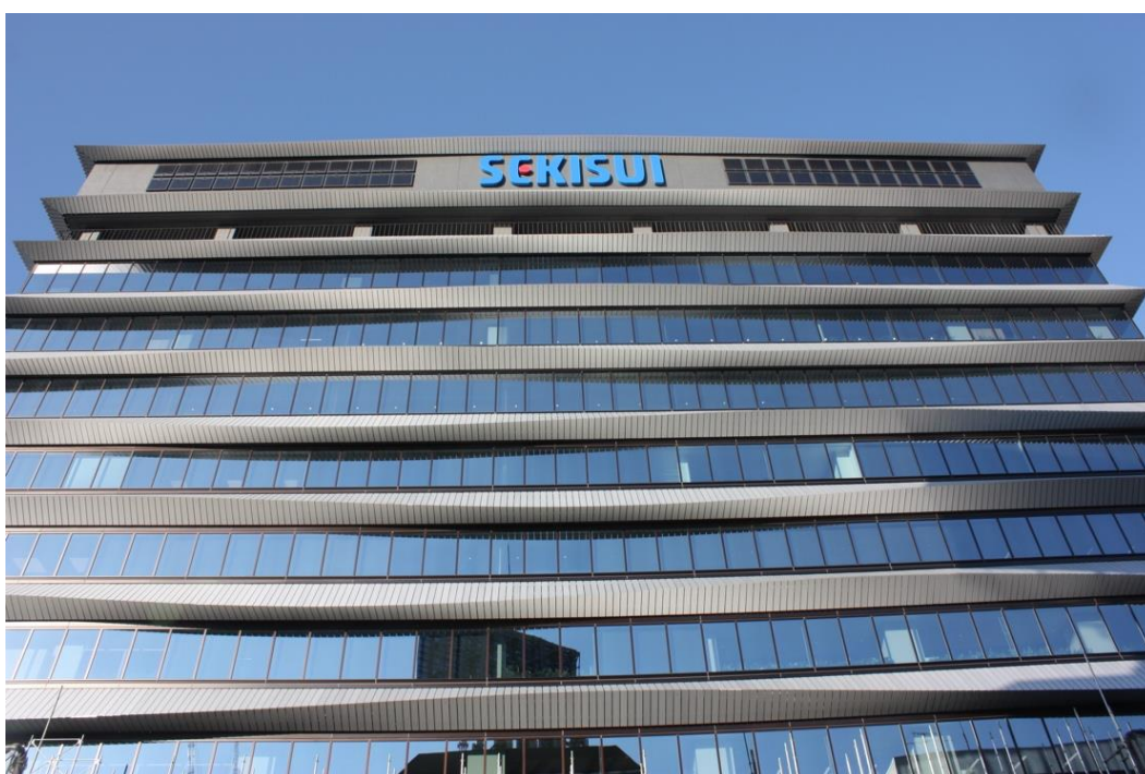
Photo 21: Wall-mounted PV system at Sekisui Chemical's Osaka Headquarters building (48 pieces of building-integrated film-type perovskite PV modules manufactured by Sekisui Chemical) in Osaka City, Osaka Prefecture, Japan
