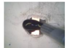
15. Sealing with silicone
