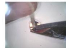
11. Cutting excess bus bar
