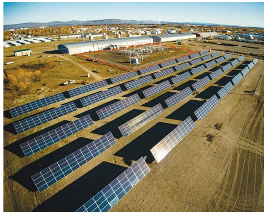
563-kW array in Fairbanks, AK
