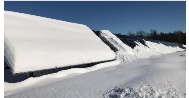
Snow covered array [Alaska, USA]
