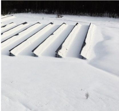
PV installation where snow cannot shed [Östersund, SE]. Image courtesy of Alexander Granlund (RISE)
