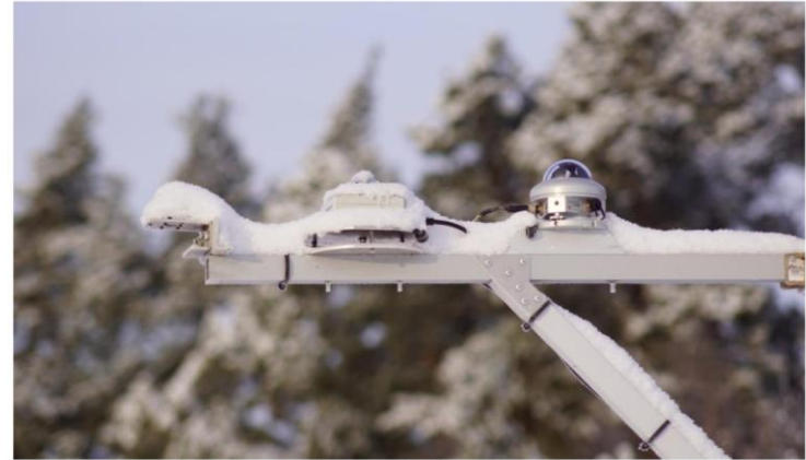
Figure 14: Photo of sensors with snow buildup and without snow buildup (built-in heating option). Photo credit Sven Ruin, TERO AB.
