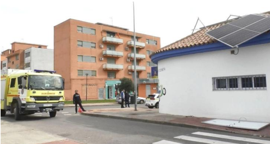
Figure 25: The structure used for solar panels installation is crucial.
