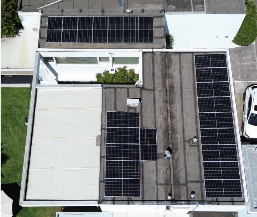
Figure 20: Solar panels installed on a mediterranean-style flat plane roof in Peñalolen, Santiago, Chile. Enough space is found available for maintenance (Source: Solar Fotovoltaica Chile).
