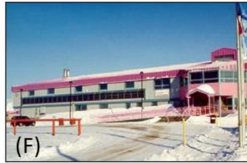
Building integrated Iqaluit, Canada
