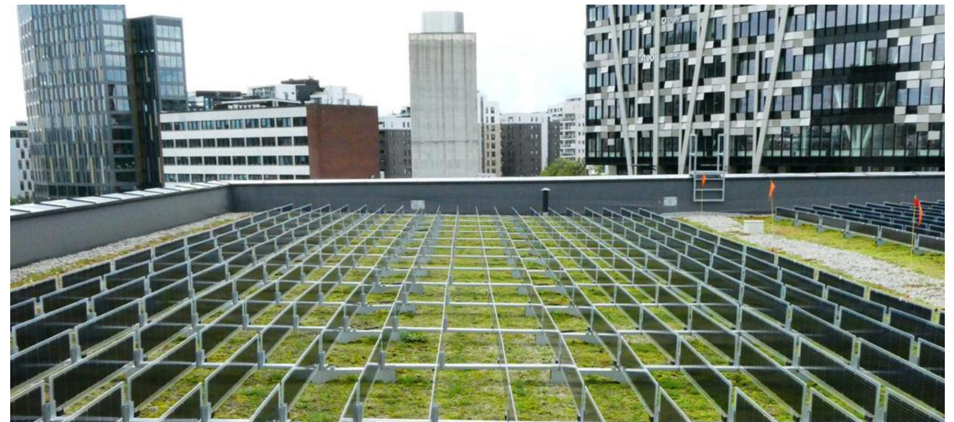
Vertical rooftop arrays in Norway. Photo credit: Over Easy Solar.
