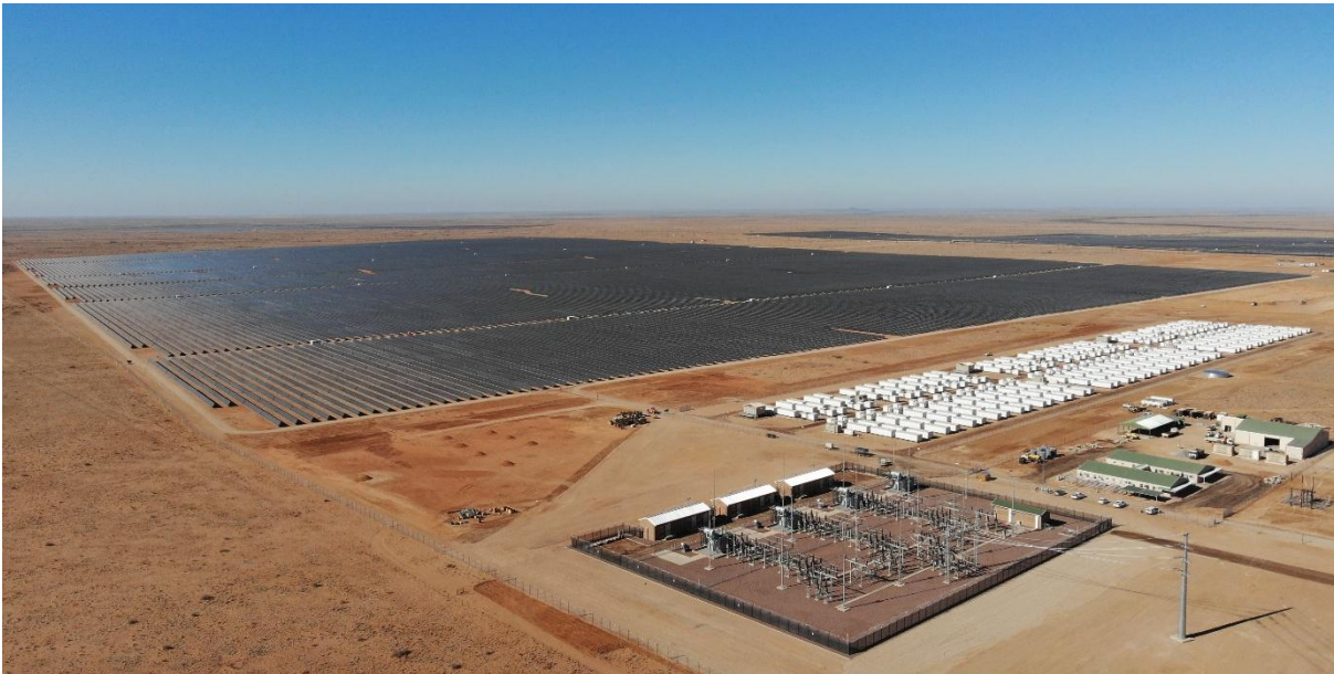
Figure 3: Overview of the utility-scale Kenhardt PV + BESS project in South Africa (Source: Scatec).
