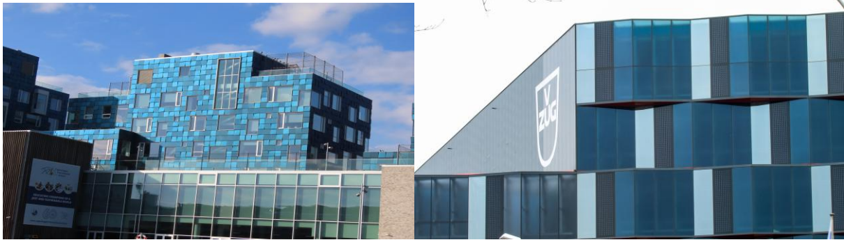
Figure 7: BIPV buildings with coloured and surface optimised modules; a) Copenhagen international school (Photo credit: Gabriele Eder/OFI), b) V-ZUG (Photo credit: © ertex solar/Dieter Moor).
