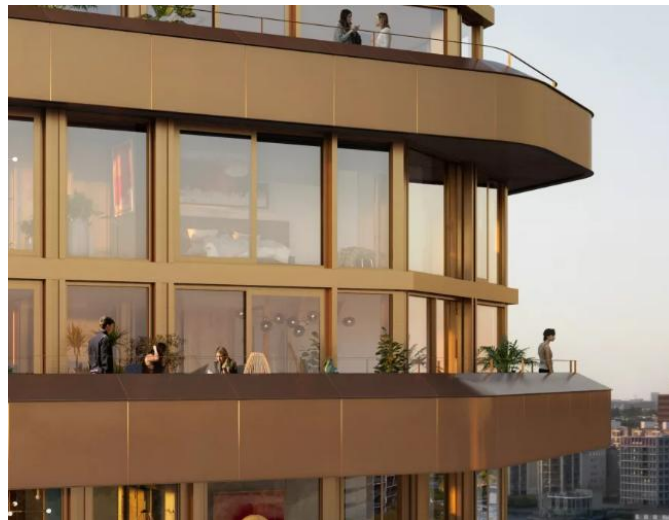
Figure 12. Close view of the parapets with customised modules in multiple orientations. (Photo credit: Kondor)
