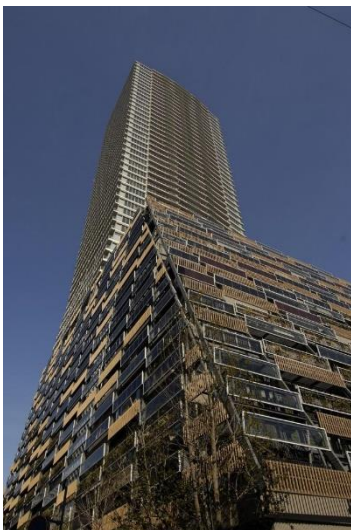
Latest example BIPV in Japan
